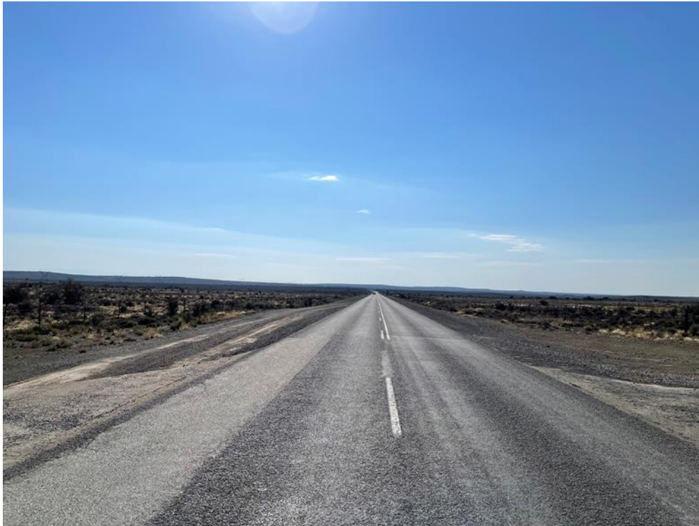
Figure 7.7 Existing Access to PTN 25 of Brits Eigendom No 374 – North Approaching
