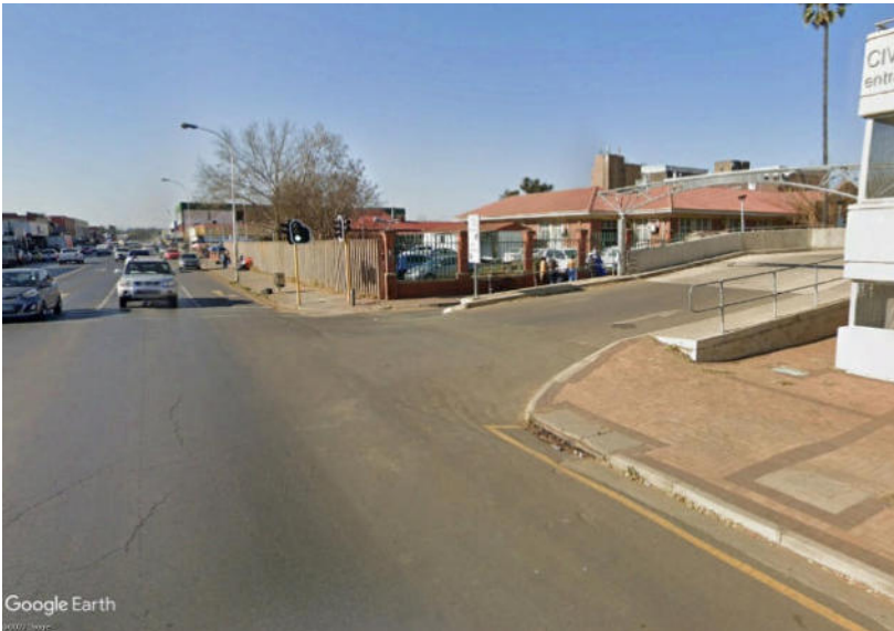
Photo 14. Photo taken on the corner of Voortrekker & Murchison Street in an Easterly direction. The site is in the top centre of the photo.
