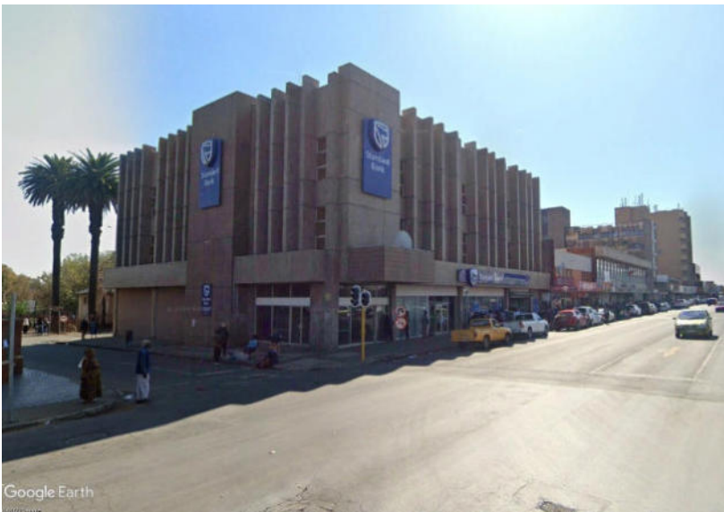
Photo 15. Photo taken on the corner of Voortrekker and Scott Street in a Northerly direction showing the street view of buildings along the rear of the site.
