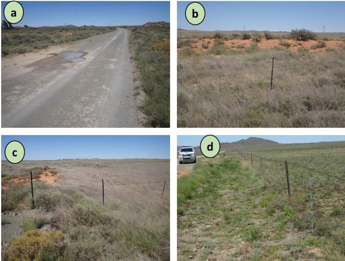
Figure 40: The road in Transect 1
