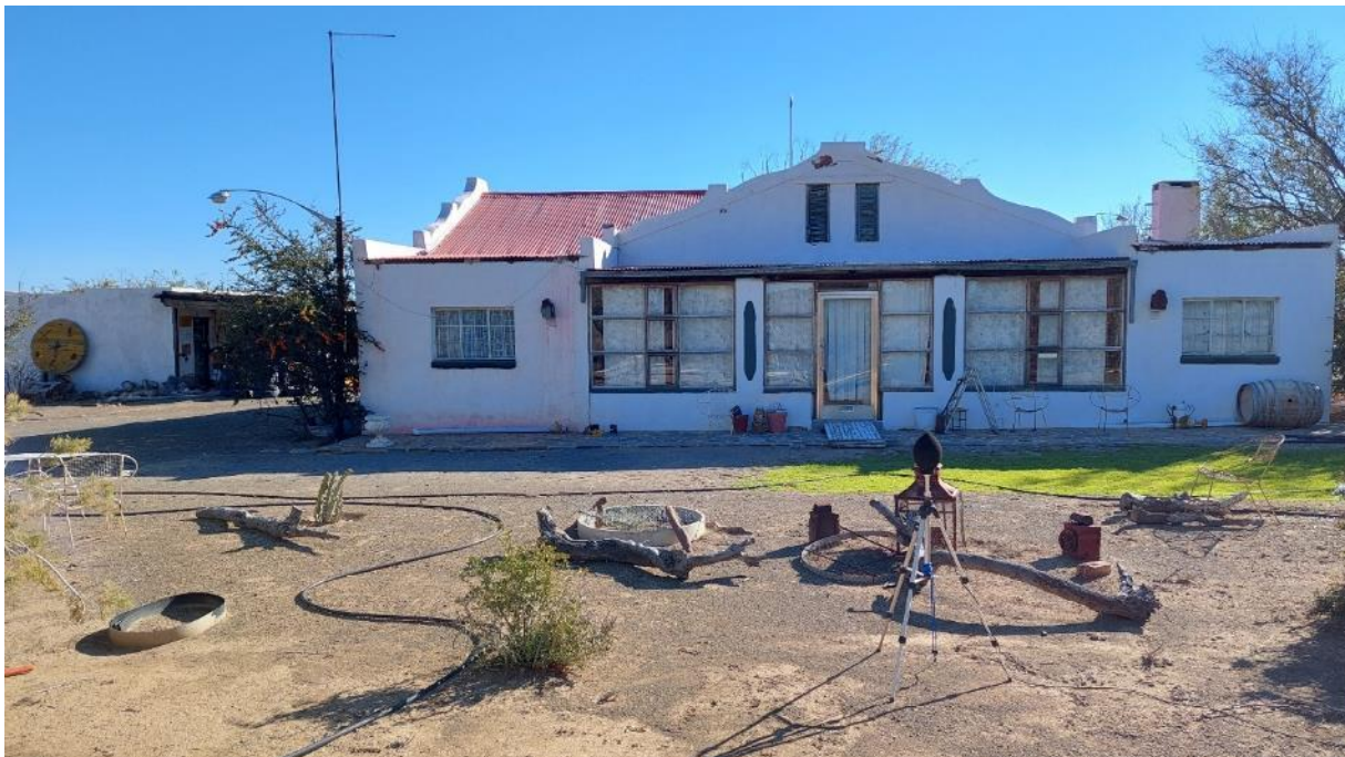
Photos E.1: Measurement location at SGEKLTSL01
