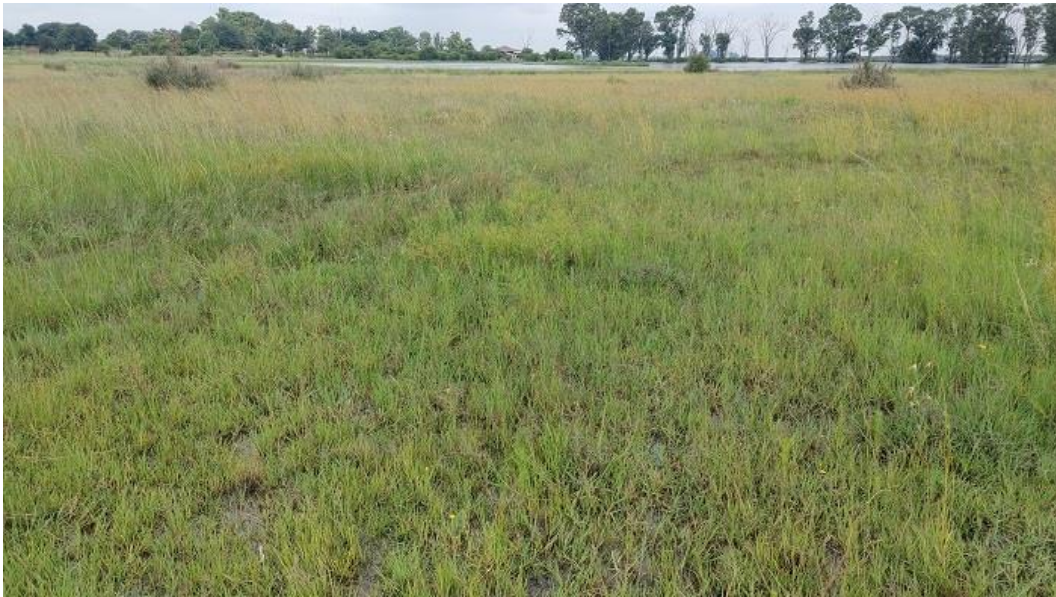
Figure 9: Two images illustrating the presence of the artificially constructed earth dam, located directly adjacent south-west of the assessment area
