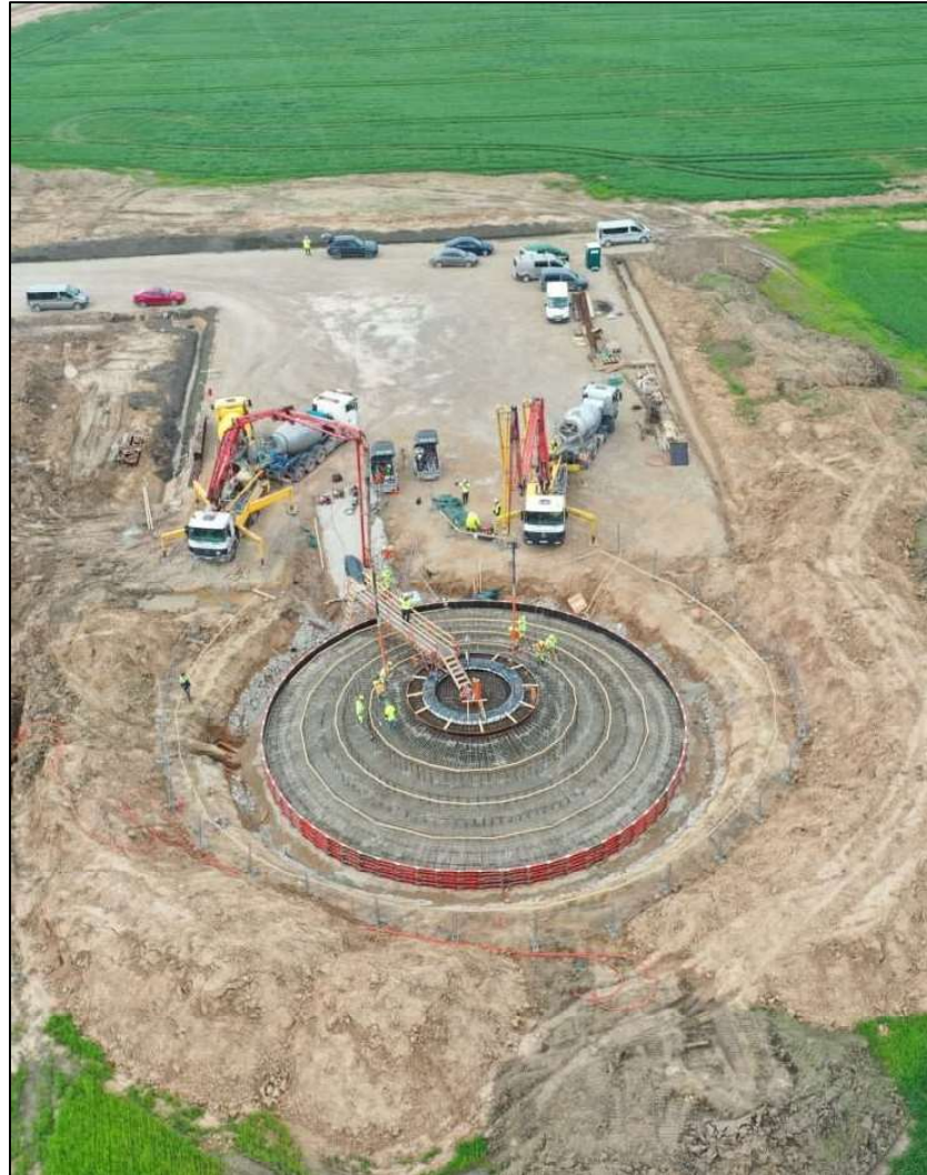
Photo 6-1 Typical Wind Turbine Foundation Construction
