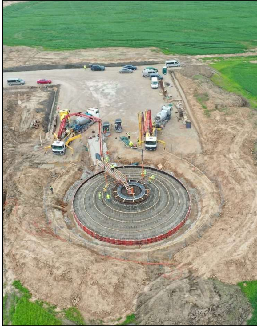
Photo 6-1 Typical Wind Turbine Foundation Construction
