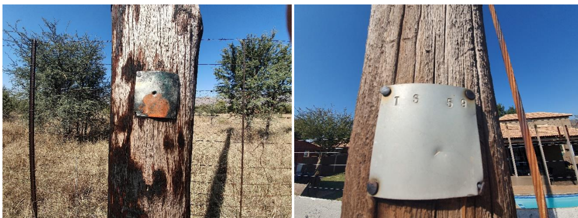
Figure 3 Poles TS 58 and TS 59 Respectively
