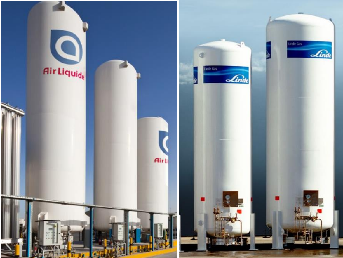
Figure 18: Cryogenic storage tanks – vertical tanks.
