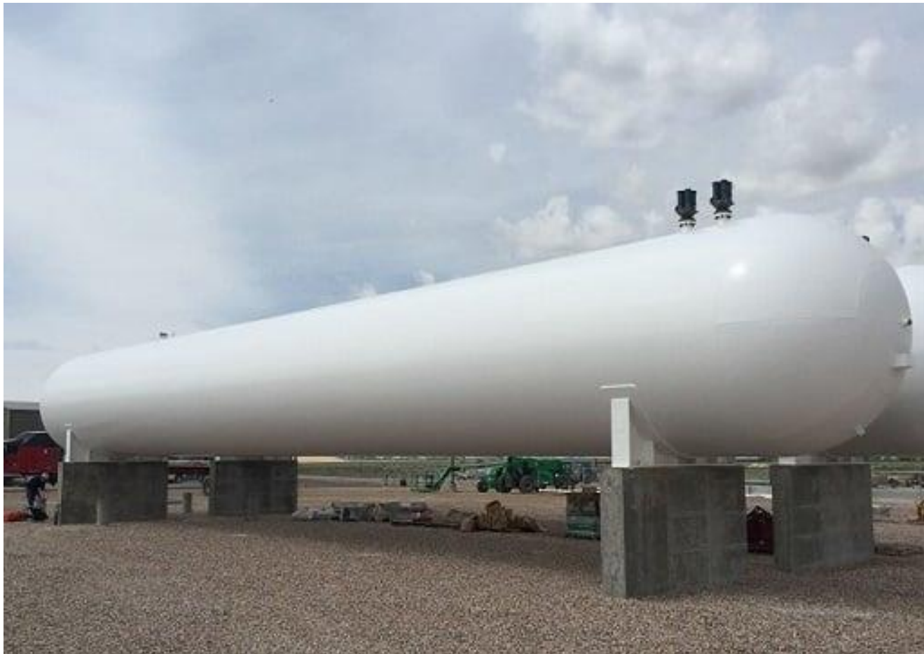
Figure 14: Bullet storage tank (ammonia storage)
