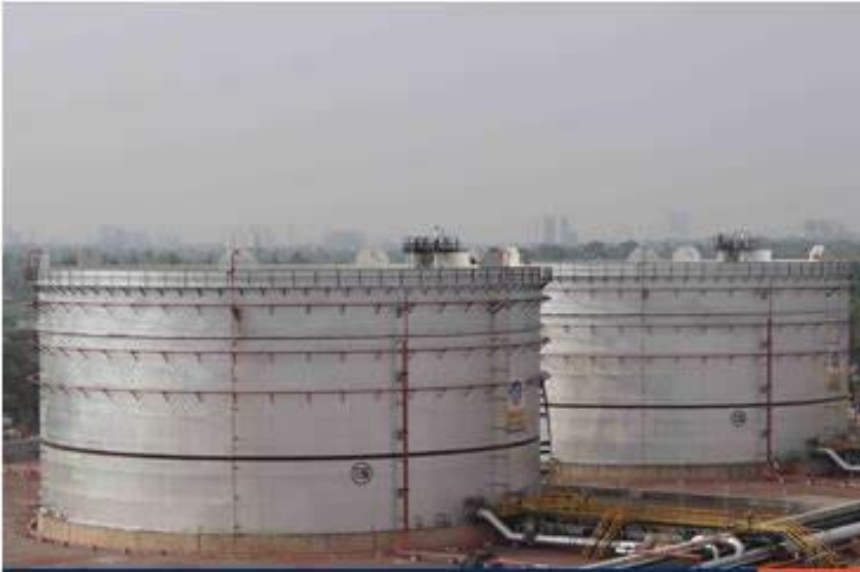
Figure 11: Double-deck floating roof storage tank
