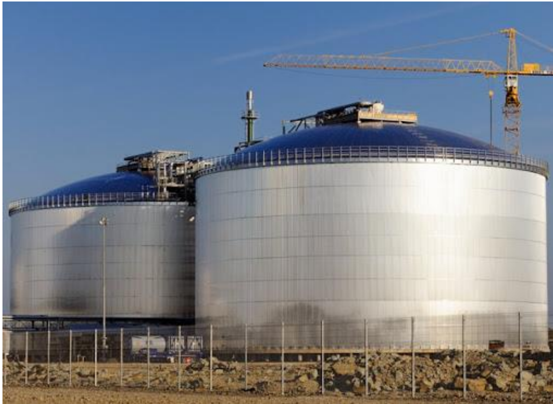
Figure 16: Cryogenic ammonia storage tanks
