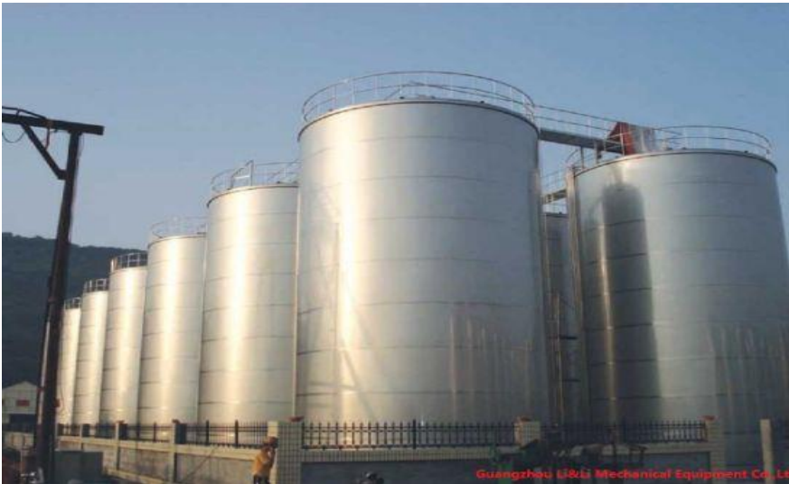
Figure 13: Stainless steel single-layered low-pressure tanks
