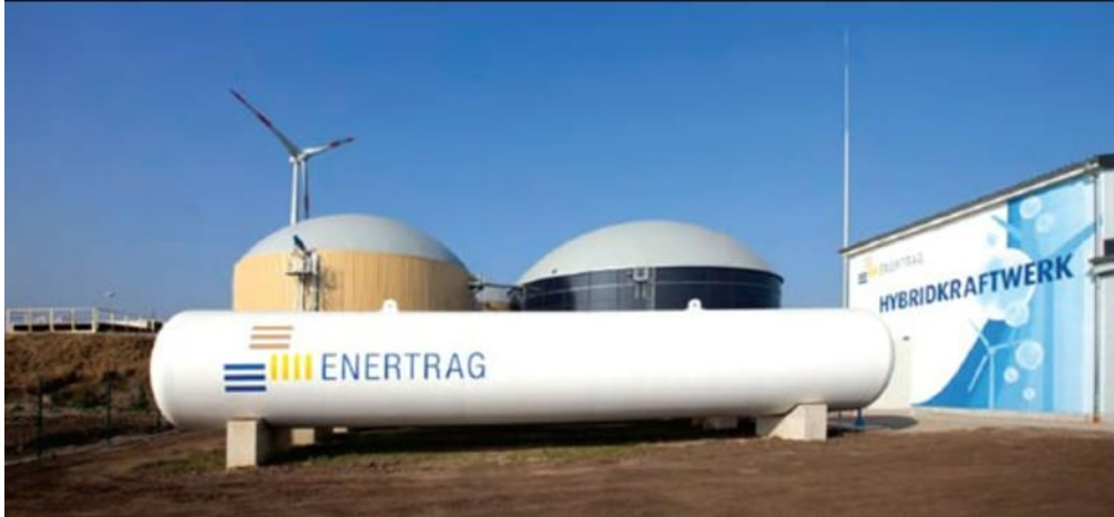
Figure 7 Compressed hydrogen tank- horizontal tank.
