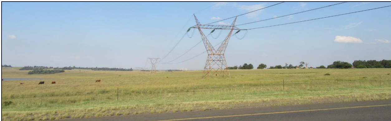
Photograph 3.10: 400 kV line crossing the N11 approximately 6 km south of Ermelo
