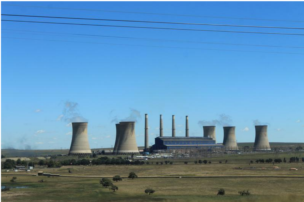
Photograph 3.1: Camden Power Station
