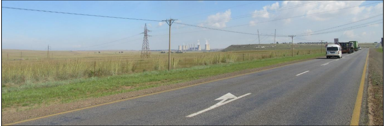
Photograph 3.9: Camden power station and power lines seen from the east from near Mooiplaas colliery on the N2
