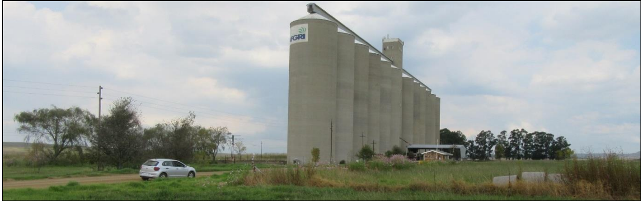
Photograph 3.4: Overvaal silo located adjacent to Richards Bay railway line
