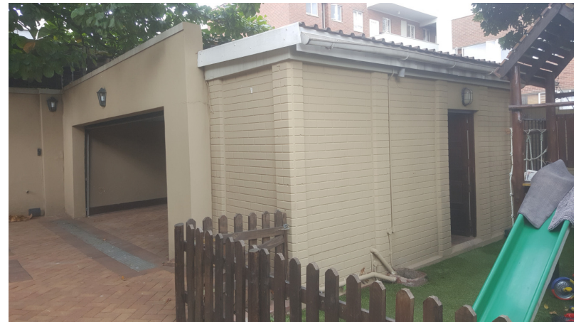
NORTH CORNER OF GARAGE AND PREFAB LAUNDRY – LAUNDRY TO BE DEMOLISHED.
