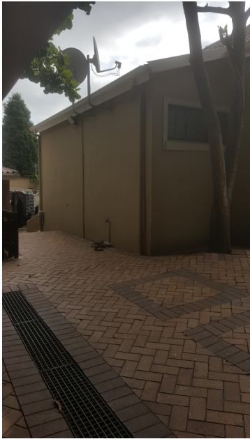
SOUTH CORNER – VIEWING SW ELEVATION MAIN BUILDING
