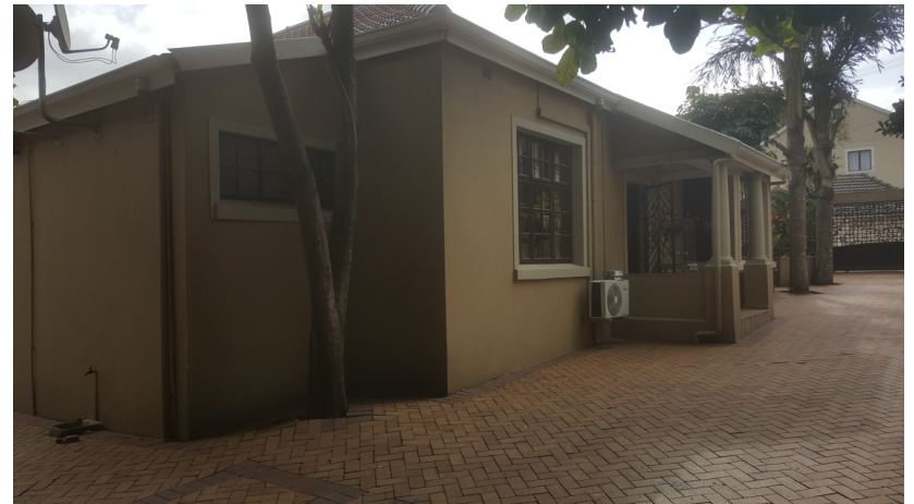
SOUTH CORNER – VIEWING SE ELEVATION - MAIN BUILDING
