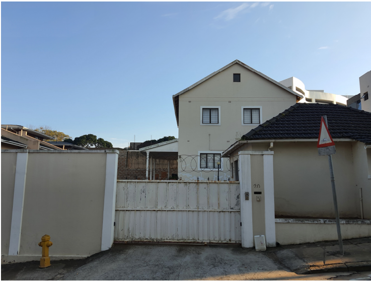
OPPOSITE NEIGHBOUR AT 20 NELSON ROAD
