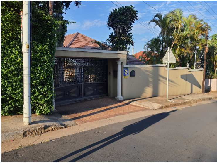
ROAD VIEW OF 21 NELSON ROAD
