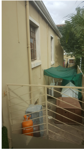
NORTH CORNER – VIEWING NW ELEVATION MAIN BUILDING
