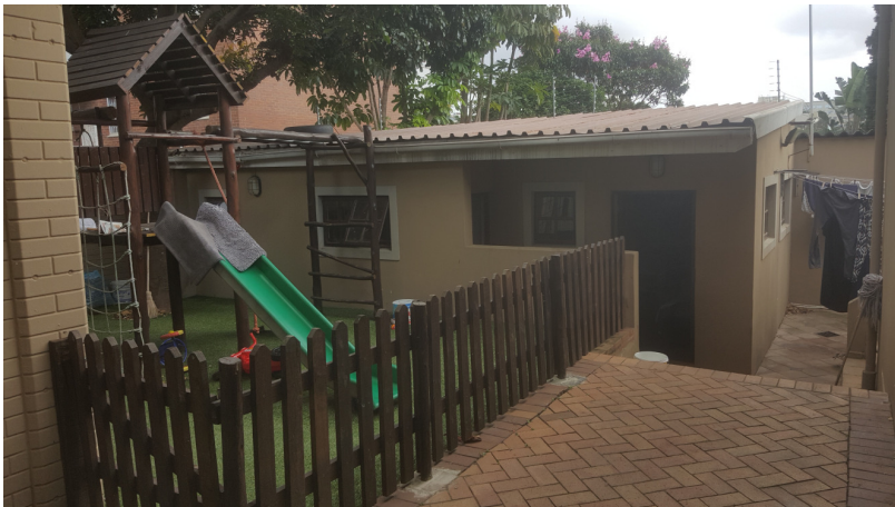
MAID'S QUARTERS / OUTBUILDING TO BE DEMOLISHED
