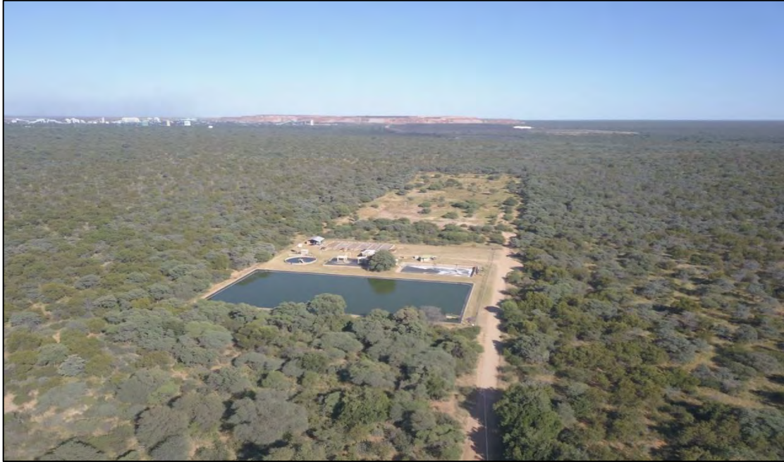
Plate 9-1: Aerial view of the Waste Water Treatment Works and associated drying beds
