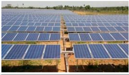
Figure 3-1: Single axis solar PV module tables raised 1.5m above ground level (to a maximum tilt height of 3m) 14
