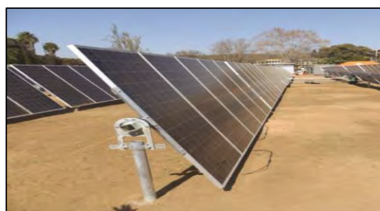
Figure 1-3: Single axis solar PV module tables raised 1.5m above ground level (to a maximum tilt height of 3m).
