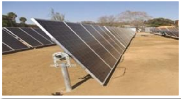
Figure 3-1: Single axis solar PV module tables raised 1.5m above ground level (to a maximum tilt height of 3m) 14
