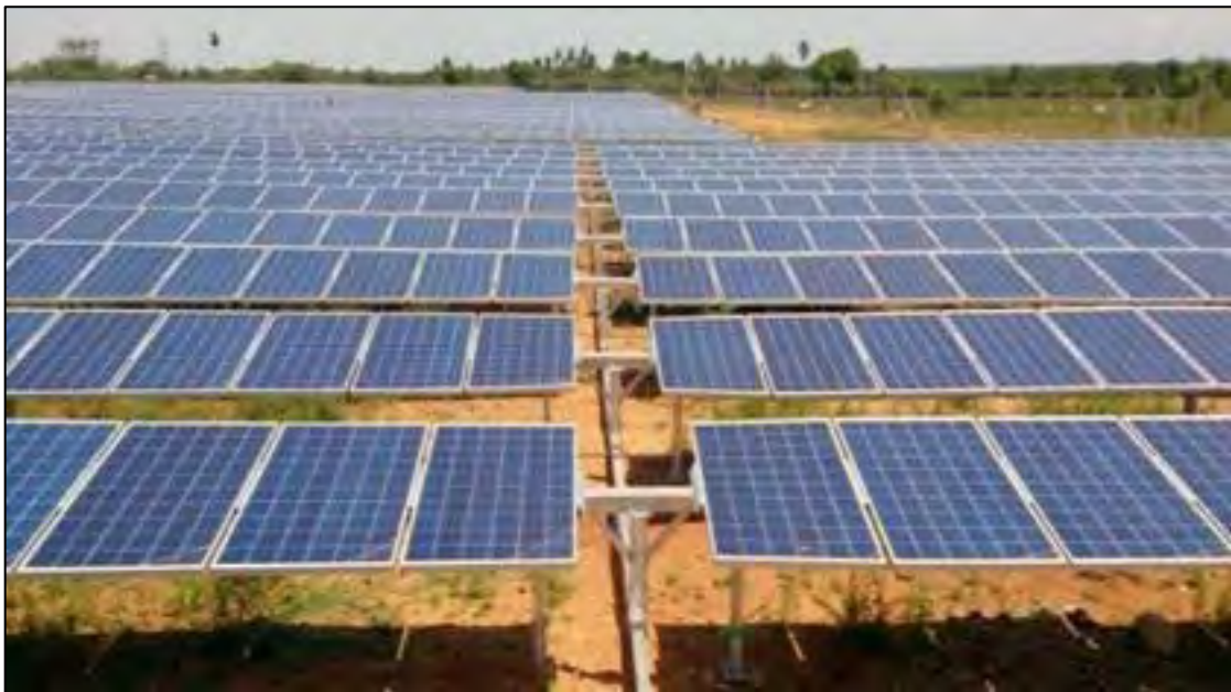
Plate 1-1: Single axis solar PV module tables raised 1.5m above ground level (to a maximum tilt height of 3m).
