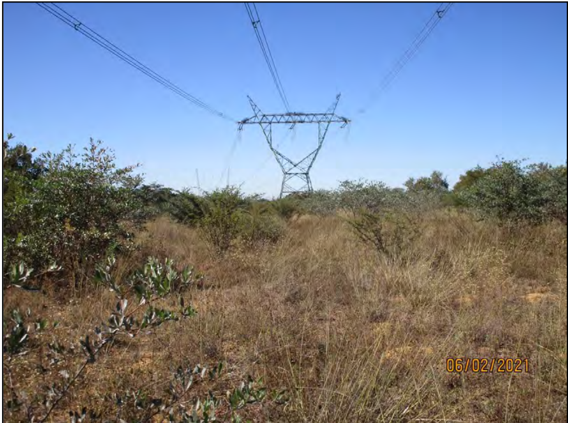
Figure 6. View of high voltage power line just east of the project area.
