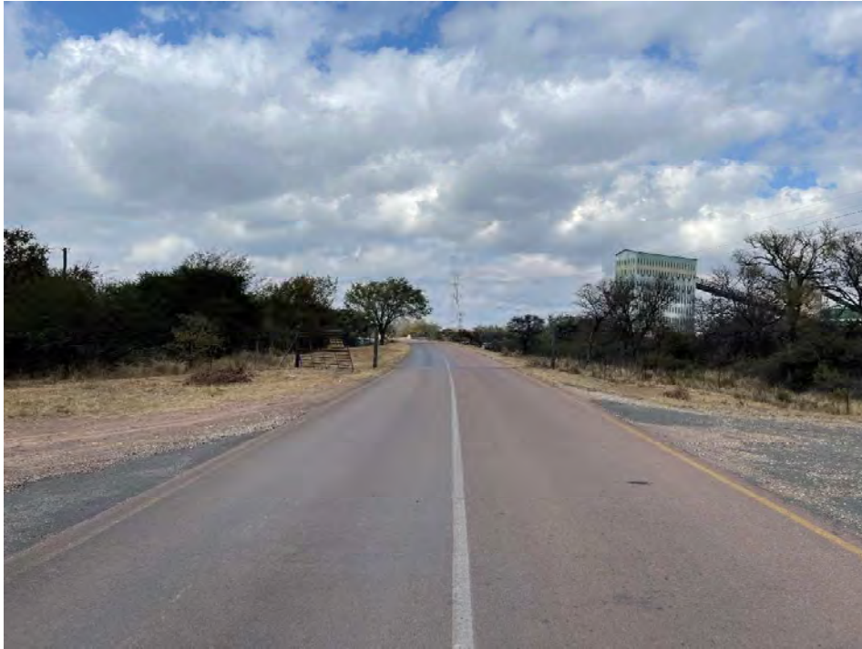
Figure 7.8 Existing Access to Lephalale Solar Project - South approaching
