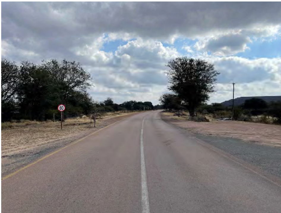
Figure 7.9 Existing Access to Lephalale Solar Project - North approaching
