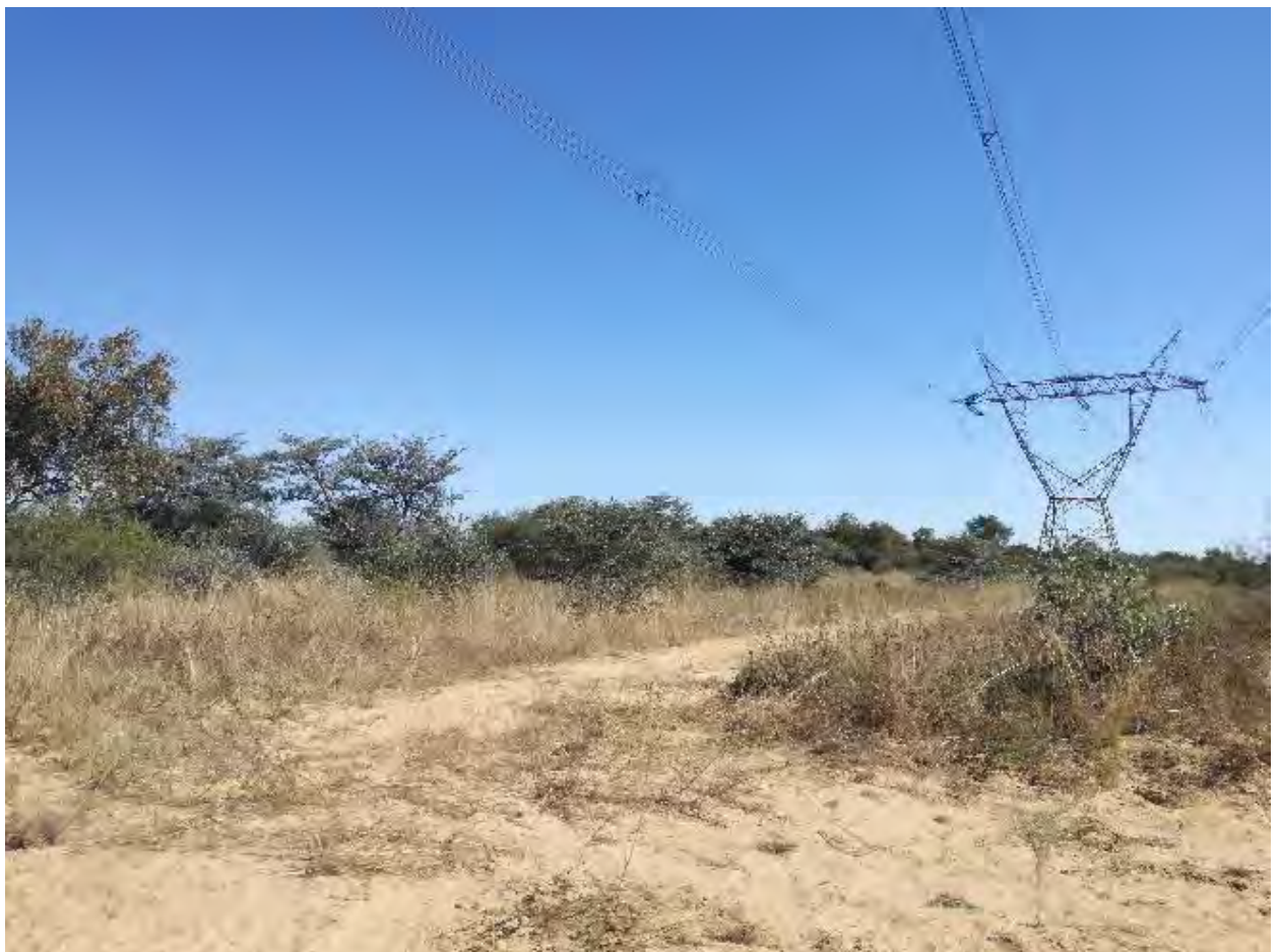
Photo 12-9: Existing Transmission Line visible from Lephalale Marapong Housing
