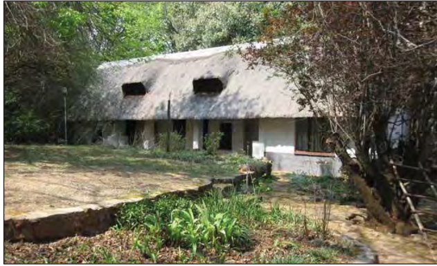
Figure 147 – Another view of the farmhouse as recorded in 2012 (Photo: Kitto & Fourie, 2012).
