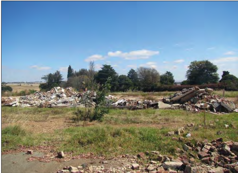
Figure 55 - General view of the demolished remains observed at site PP 07.
