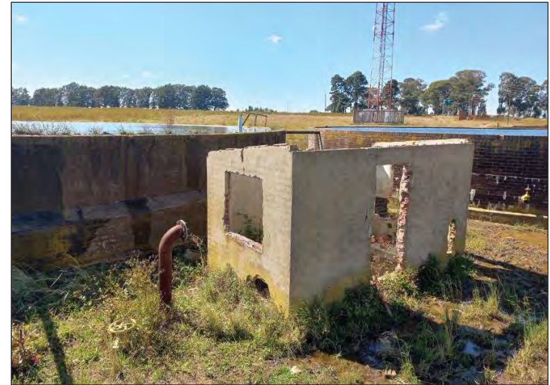
Figure 180 - General view of the site showing sections of the two reservoirs in the back with one of the associated brick buildings visible in the foreground.
