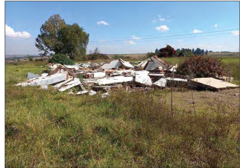
Figure 178 - General view of the demolished structure at site PP 43.
