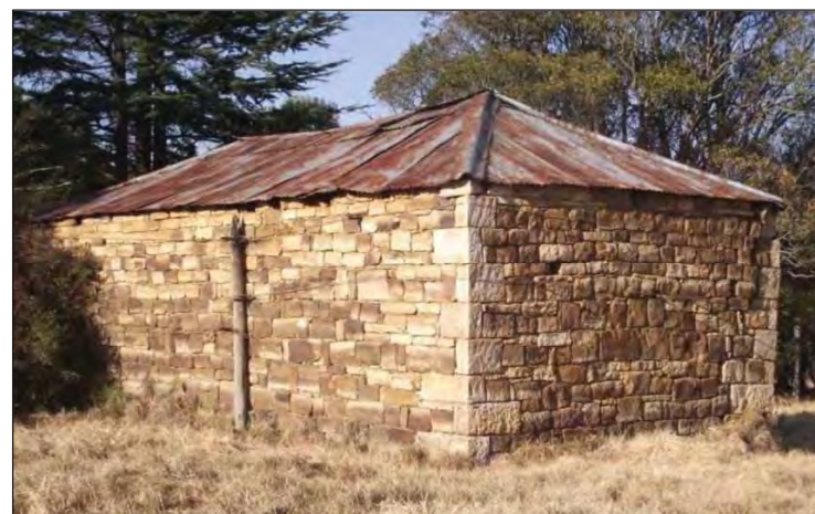
Figure 59 – The sandstone storeroom as recorded during 2012 (Photo: Kitto & Fourie, 2012).
