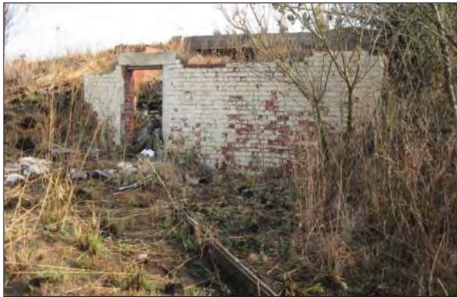
Figure 122 - Remains of the building at the Sunbury Railway Station as recorded in 2012 (Photo: Kitto & Fourie, 2012).
