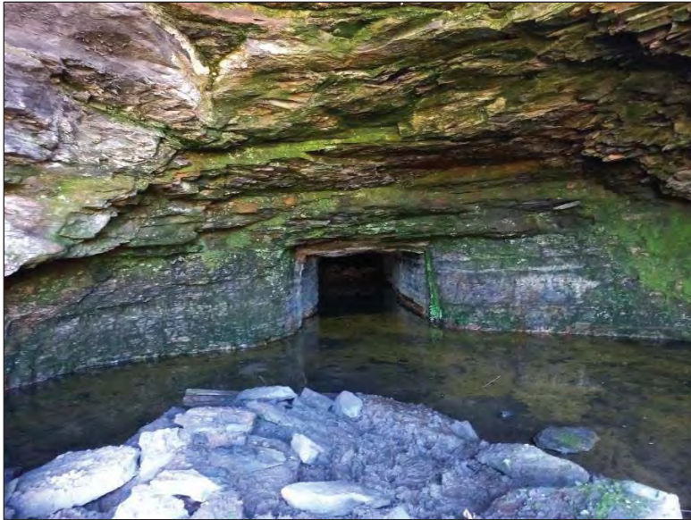
Figure 101 - Interior view of the shaft as recorded during the recent fieldwork.
