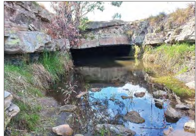
Figure 84 – Closer view of the shaft entrance at PP 13 as recorded during the recent fieldwork.
