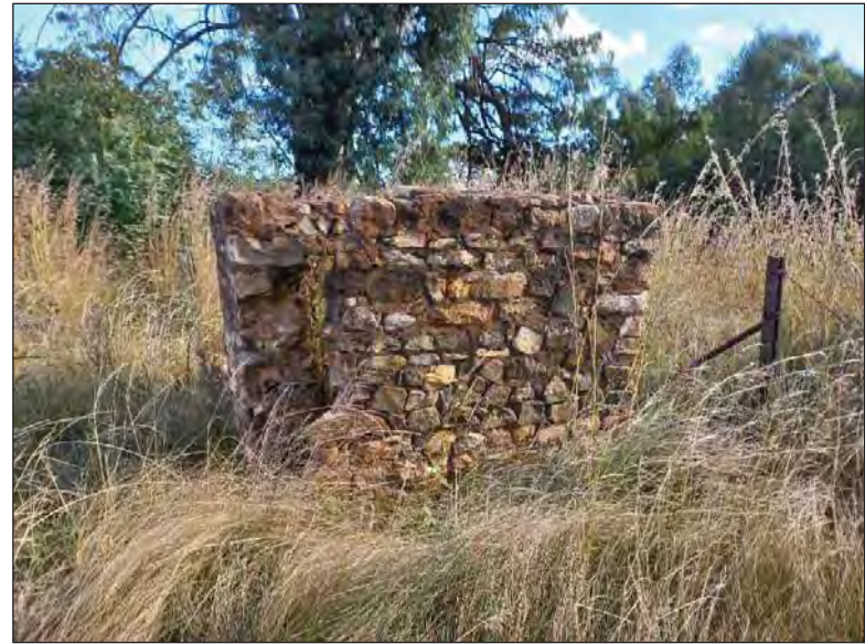
Figure 176 – General view of the stone structure at site PP 41.
