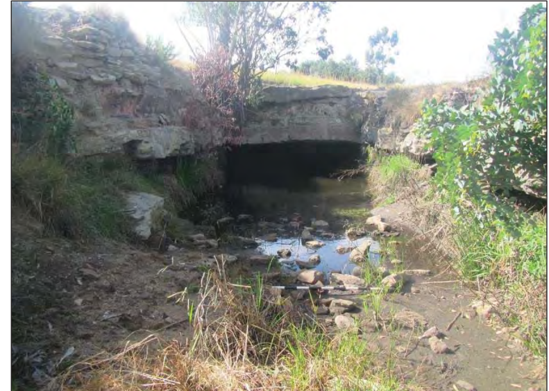
Figure 83 – General view of the shaft entrance at PP 13 as recorded during the recent fieldwork. The scale is in 10cm increments.
