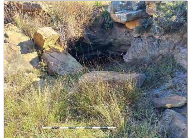
Figure 167 - View of the entrance to the abandoned coal mine shaft at PP 36. The scale is in 10cm increments.
