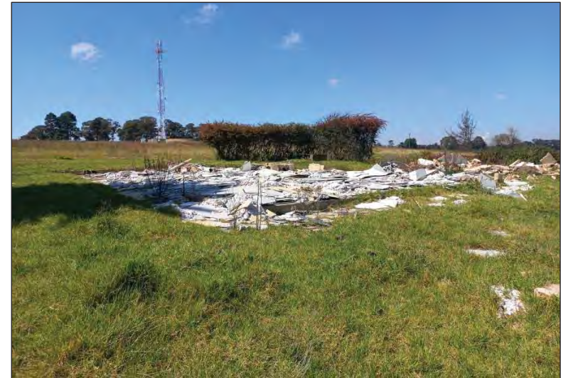
Figure 182 - General view of the demolished structure at site PP 45.
