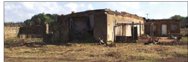
Figure 48 - Close-up view of a dwelling addition as recorded in 2012 (Photo: Kitto & Fourie, 2012).
