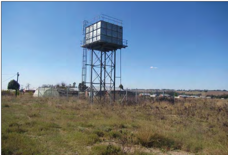
Figure 110 – The new steel reservoir that was built near site PP 20. This steel reservoir is associated with the Phumulani Agri-Village.
