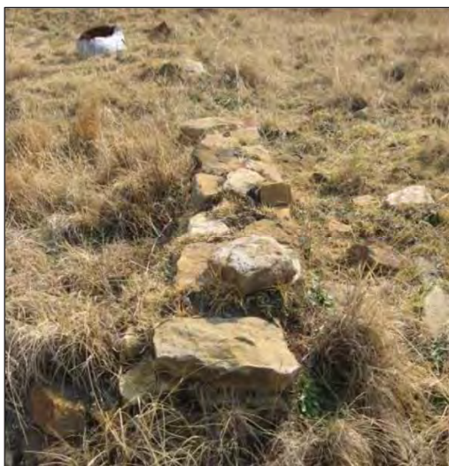
Figure 129 - Foundation of the homestead as recorded in 2012 (Photo: Kitto & Fourie, 2012).
