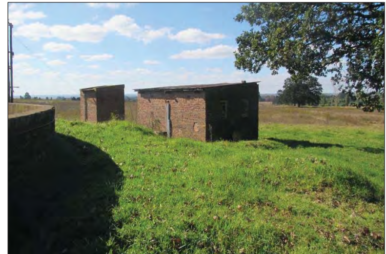
Figure 173 – A section of the reservoir is visible on the left, with the two associated brick structures located in the back.
