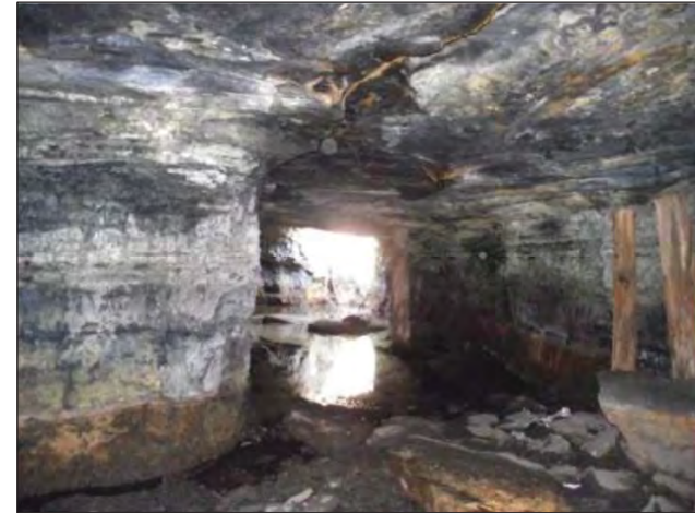
Figure 78 - Interior view of mine shaft as recorded in 2012 (Photo: Kitto & Fourie, 2012).
