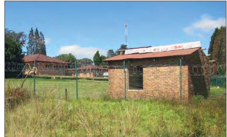
Figure 165 - General view of the two brick houses (visible in the background) with an associated smaller brick building in the foreground.
