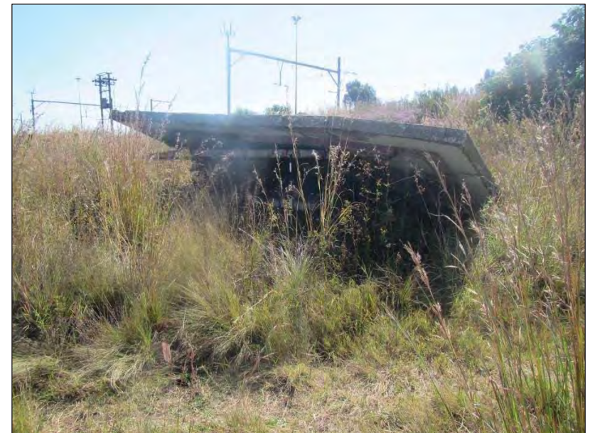
Figure 123 - The collapsed remains of the building associated with the Sunbury Railway Station as recorded during the recent fieldwork.
