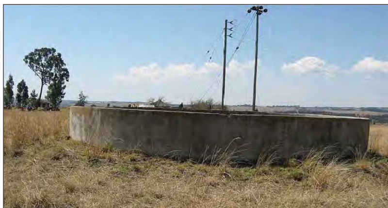
Figure 107 – General view of the brick and cement dam as recorded during the fieldwork undertaken in 2012 (Photo: Kitto & Fourie, 2012).
