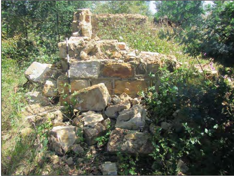
Figure 65 – Another view of the structure as recorded in 2021. The scale is in 10cm increments.
