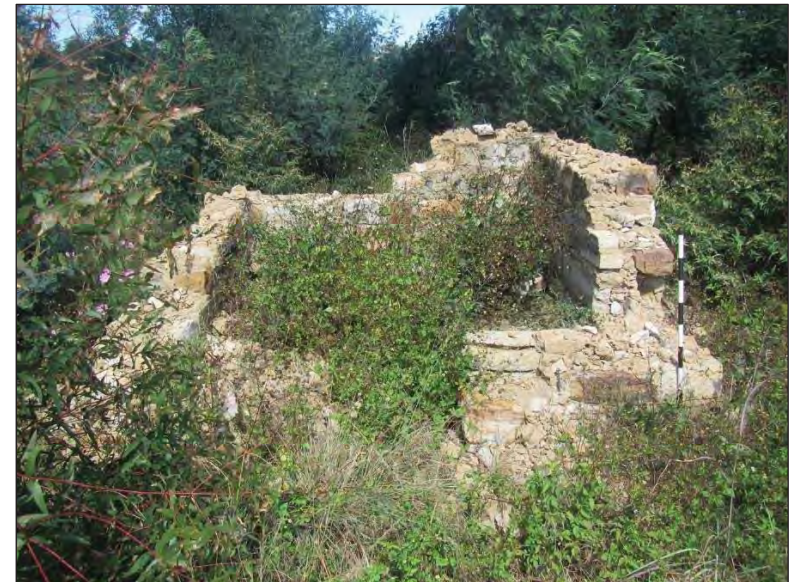
Figure 64 - View of the front of the structure as recorded in 2021. This view of the structure shows the same façade as the one that was taken in 2012 above. A comparison of the two photographs clearly show the level of deterioration at the site. The scale is in 10cm increments.
