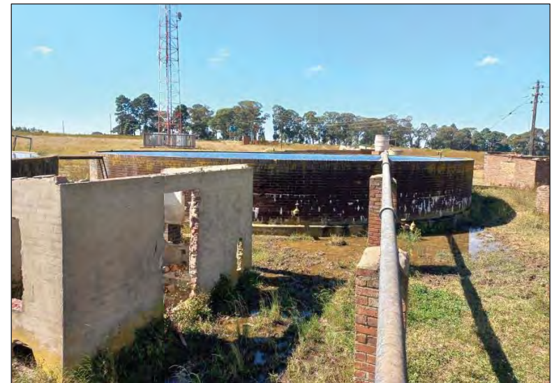
Figure 181 – Another view of the site showing a reservoir and its associated buildings and structures. 6.2.45 PP 45
