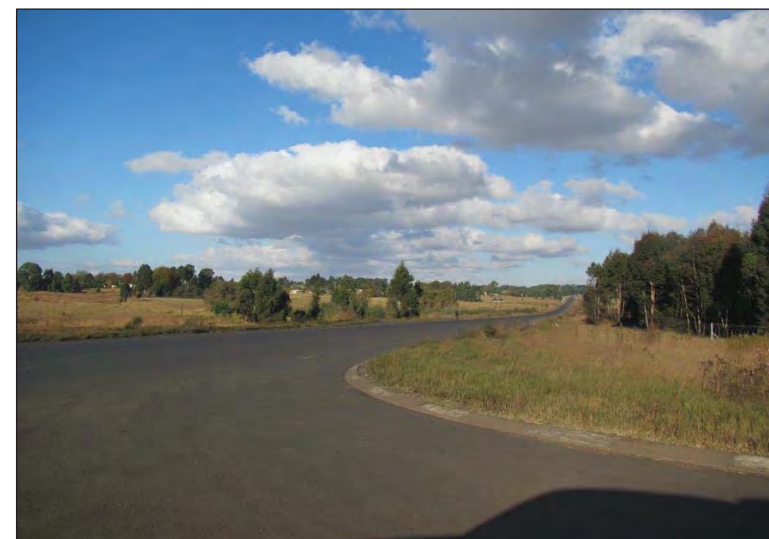
Figure 8 – General view of the N4. This road provides access to the eastern section of the project area.
