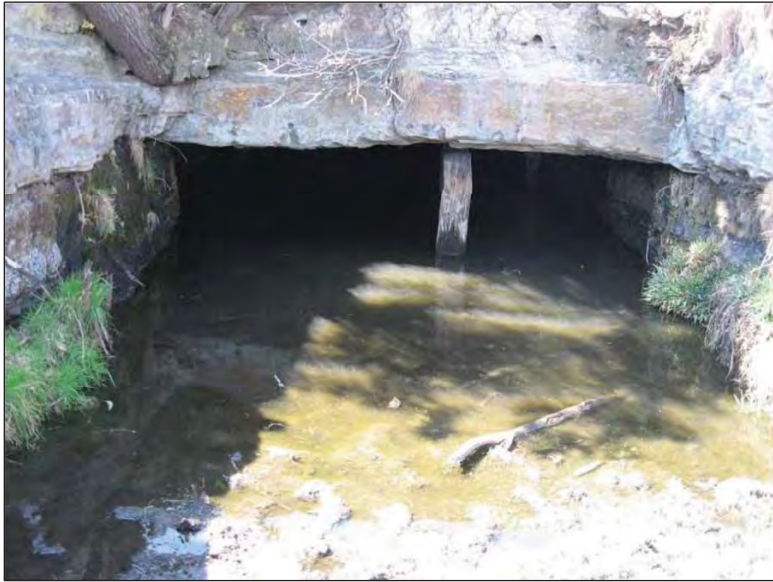
Figure 82 - Close-up view of the shaft entrance as recorded in 2012 (Photo: Kitto & Fourie, 2012).
