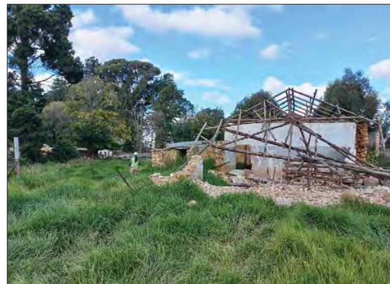
Figure 153 - View of the stone building with collapsed roof. The scale is in 10cm increments.
