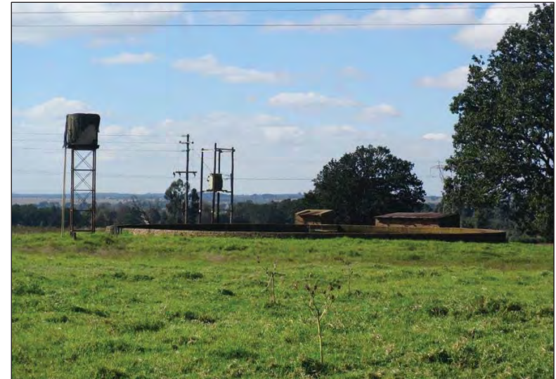
Figure 172 - General view of the reservoir and buildings at site PP 39.
