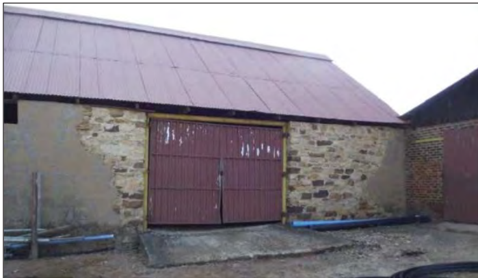
Figure 52 – General view of the large storeroom as recorded in 2012 (Photo: Kitto & Fourie, 2012).
