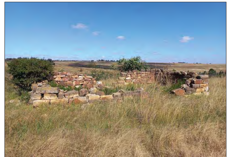
Figure 136 – Closer view of the sandstone building as recorded during the recent fieldwork.
