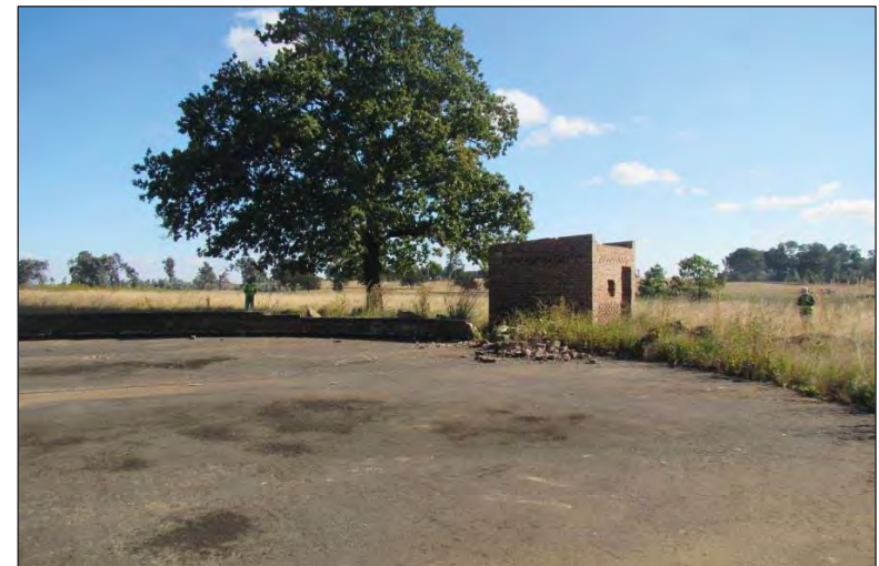
Figure 171 – Another view of the site showing a section of the reservoir in the foreground with the brick building in the back.
