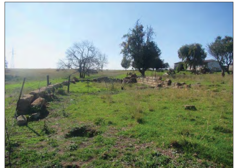
Figure 76 - General view of the stone kraal. The scale is in 10 cm increments.
