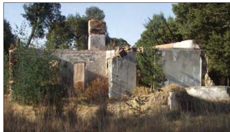
Figure 58 – General view of the farmhouse as recorded in 2012 (Photo: Kitto & Fourie, 2012).
