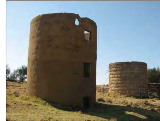
Figure 72 – The two silos from site PP 10 as recorded in 2012 (Photo: Kitto & Fourie, 2012).
