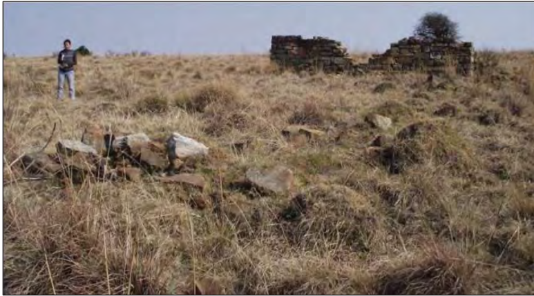
Figure 134 – Another view of the site as recorded in 2012. This image depicts the remains of walls associated with the building (Photo: Kitto & Fourie, 2012).
