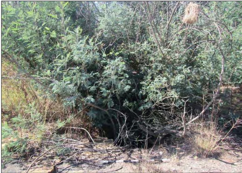
Figure 80 – Closer view of the entrance to the shaft as recorded during the recent fieldwork. As can be seen, the shaft entrance is completely overgrown. The scale is in 10cm increments.
