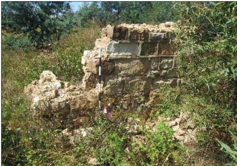
Figure 66 – Another view of the structure as recorded in 2021. The scale is in 10cm increments.
