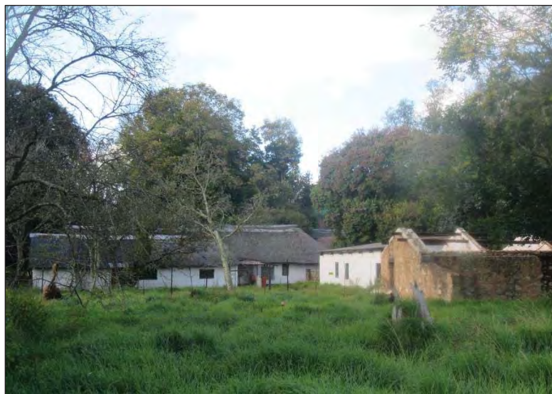
Figure 152 - General view of the farmstead at site PP 30 as recorded during the recent visit to the site. The thatched-roof farmhouse can be seen in the background on the left.
