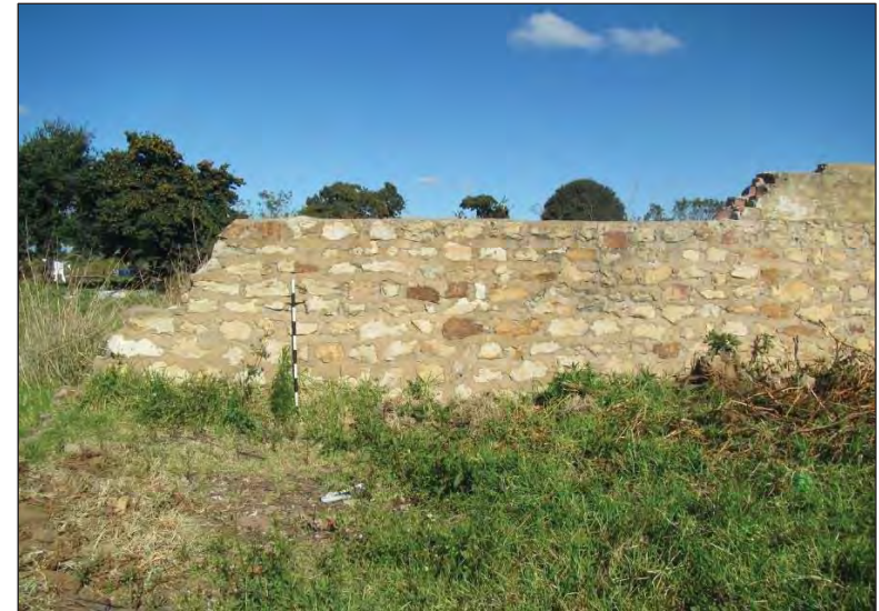
Figure 50 – Closer view of a section of walling from the kraal. The scale is in 10cm increments.
