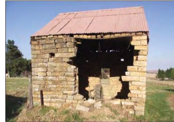
Figure 53 – The dilapidated square structure as recorded in 2012. This building was constructed of sandstone (Photo: Kitto & Fourie, 2012).
