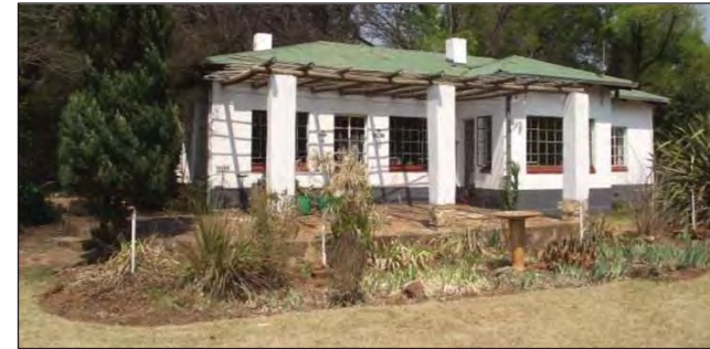
Figure 150 - Second farmhouse, the original building (Photo: Kitto & Fourie, 2012).
