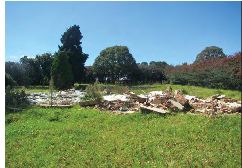
Figure 163 - General view of the demolished structure at PP 34.
