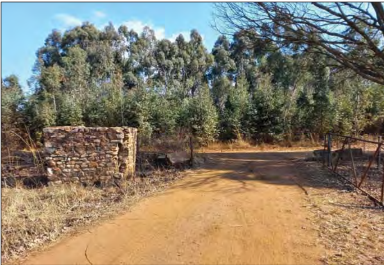
Figure 7 - View of the remains of the stone structure at PP 41 as taken on 16 July 2021.
