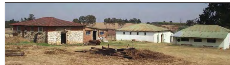
Figure 26 - Pigsty and two sheds/storerooms as recorded in 2012 (Photo: Kitto & Fourie, 2012)
