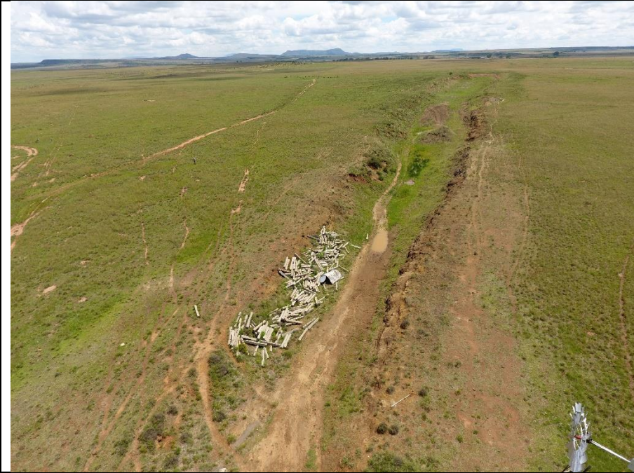
Aerial view of the existing borrow pit showing the flat topography of the surrounding area. The borrow pit strikes SW-NE. Date: January 2021.
