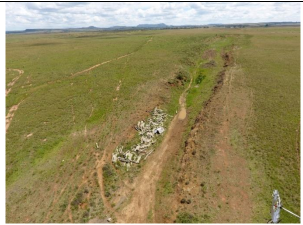
Figure 10: Aerial photograph of the existing old borrow pit striking SW-NE.
