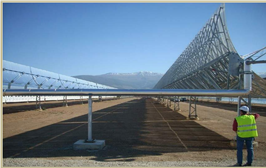
Figure 5-10: Crossover Pipe (Flagsol, 2011)
