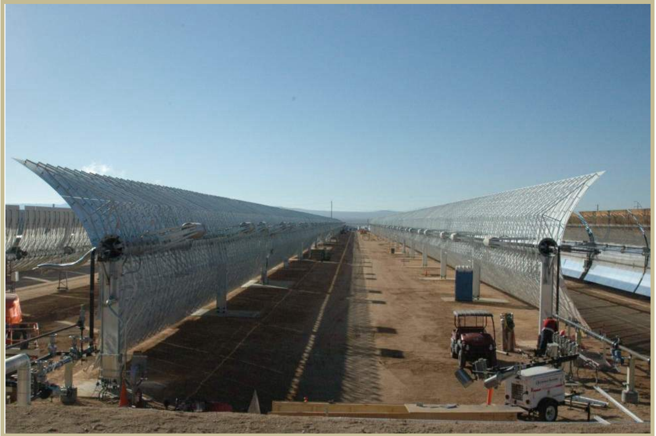
Figure 5-3: HelioTrough® Collectors installed at Kramer Junction (California /USA) (Flagsol, 2011)
