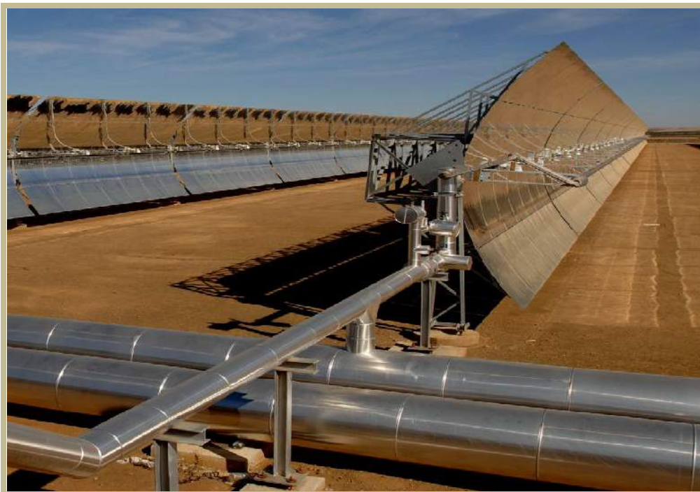
Figure 5-9: Interconnecting Piping (Flagsol, 2011)
