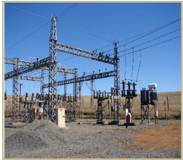
Figure 4-18: Typical outdoor high strung busbar substation (EON, 2011)
