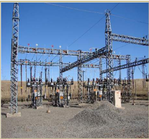
Figure 4-18: Typical outdoor high strung busbar substation (EON, 2011)
