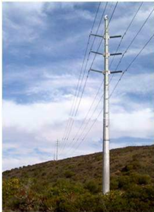
Figure 4-16: Monopole double circuit 132kV Line
