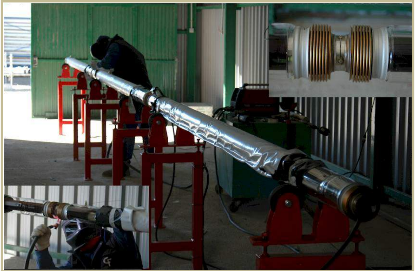
Figure 5-6: Pre Assembly of HCE elements (Flagsol, 2011)
