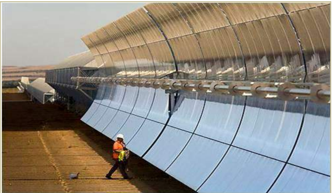
Figure 4-4: Photograph of existing parabolic trough infrastructure in Spain (Flagsol, 2010)
