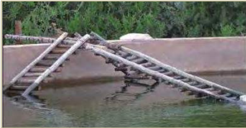
Figure 6-18: A ladder structure used to raptor-proof a reservoir
