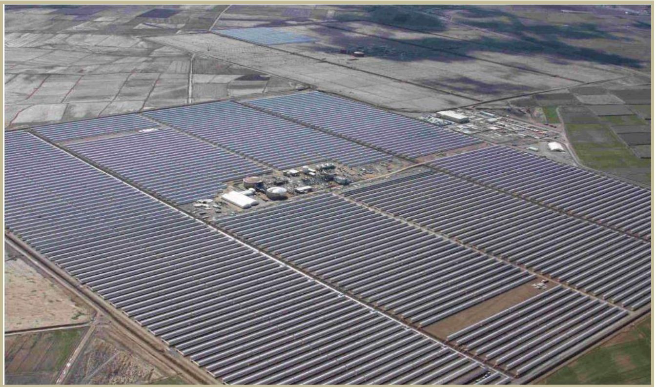
Figure 4-3: Photograph of existing parabolic trough facility in Spain (Flagsol, 2010)
