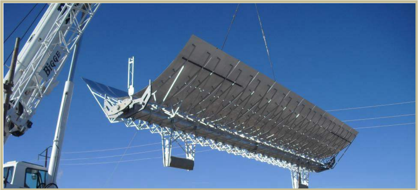
Figure 5-4: HeliTrough® SCE with main components during site erection (Flagsol, 2011)
