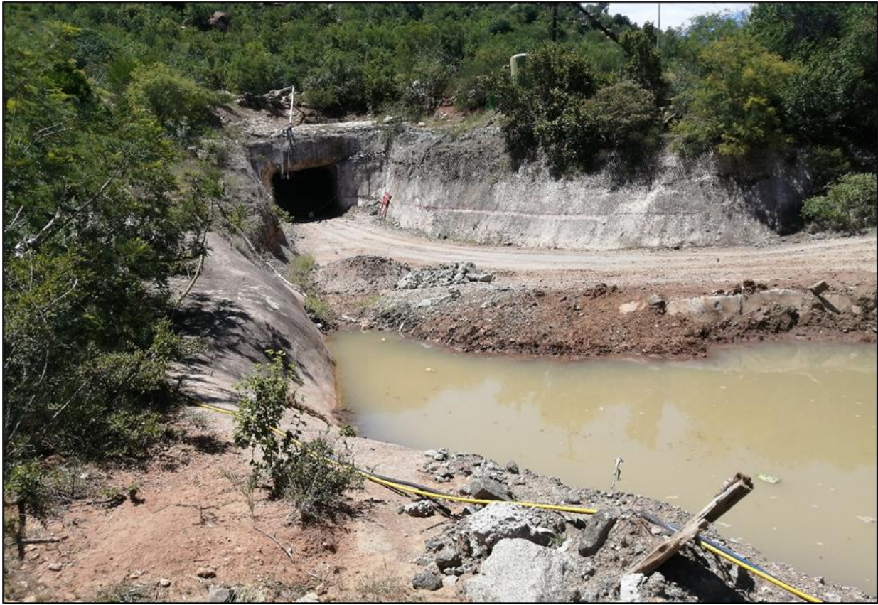
Figure 21: View of a mine adit from within the study area, that is reinforced with concrete and appears to be still in use today
