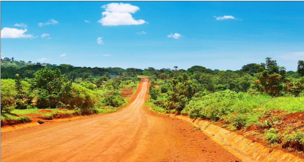
Figure 3: Typical untarred road surface
