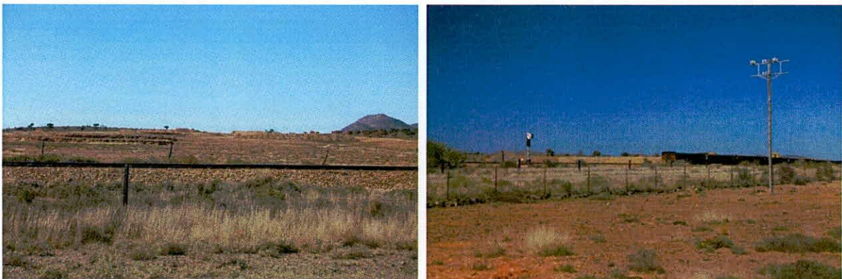
Figure 11: The railway infrastructure parallel to the R338 servicing the PPC Quarry.
