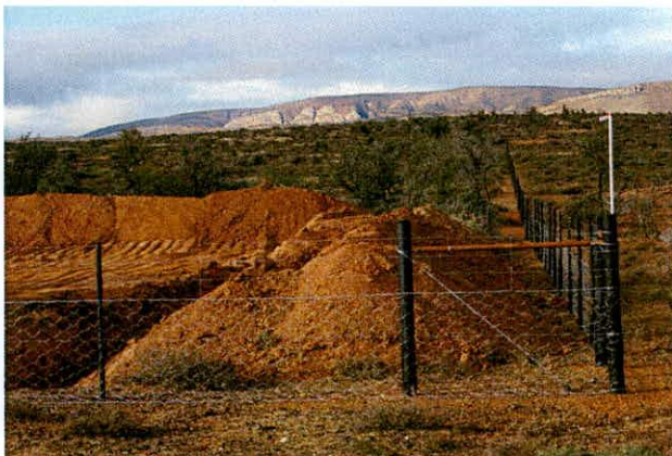
Figure 8: Topsoil is firstly stripped off and stacked aside for later rehabilitation.
