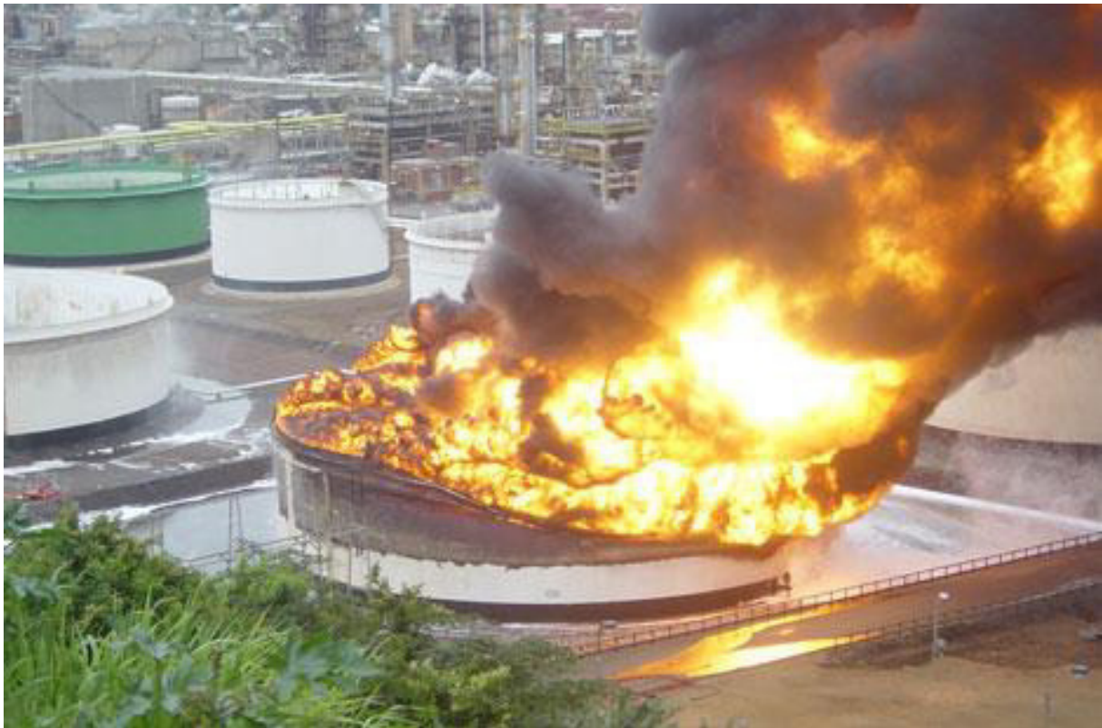
Figure 4-2: Tank-top fire at the Engen refinery caused by lightning
