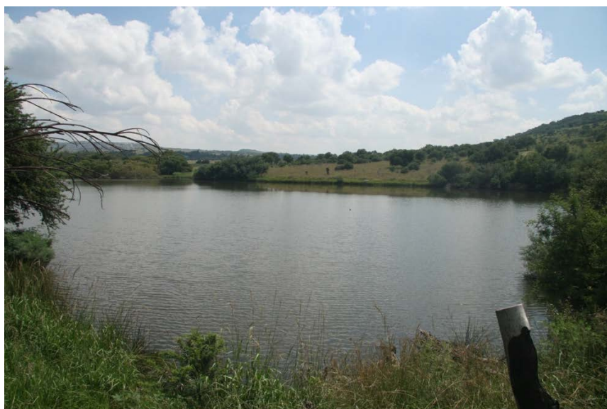
Figure 21. Dam in the Kraalkopspruit.
