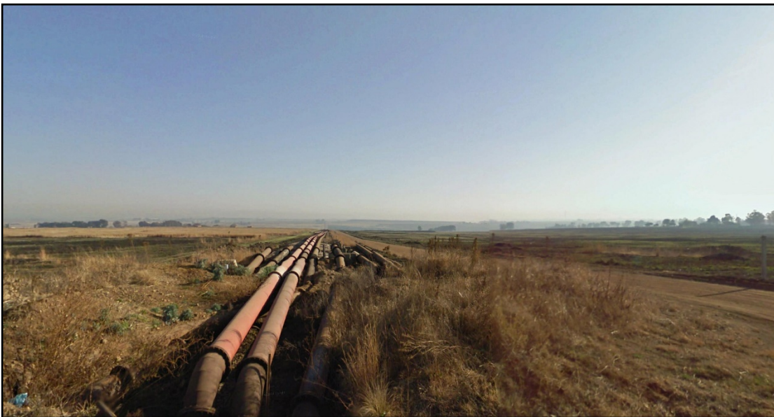
Figure 44: Existing slurry pipeline near the R23 arterial road.
