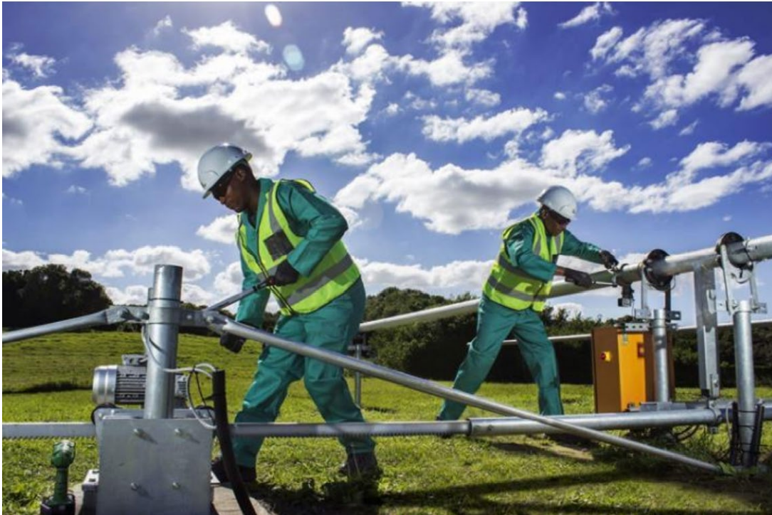
Figure 2: Single Axis Tracking for Panel Mounting
