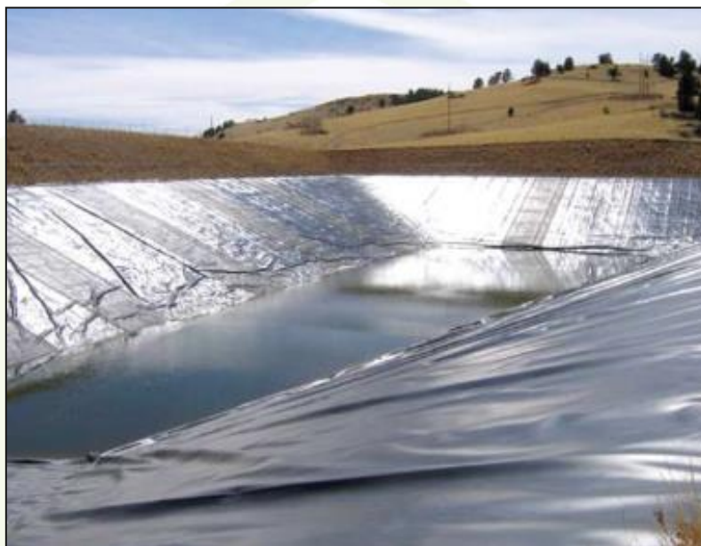
Figure 3-11: Lined PCD illustration
