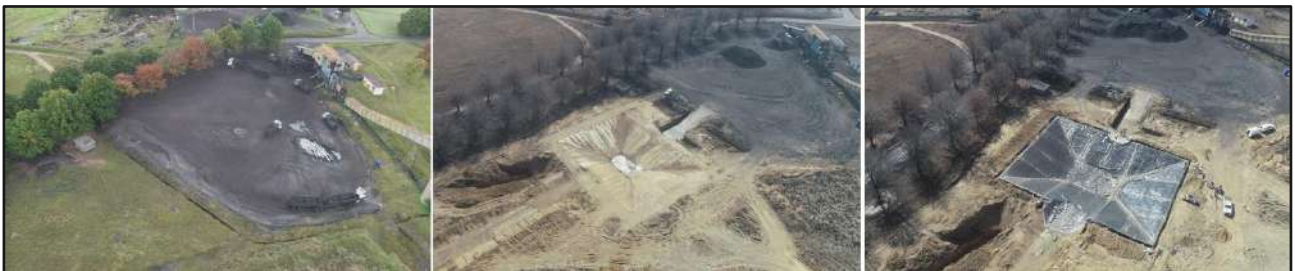
Figure 2-6: Typical lined pollution control dam (PCD)
