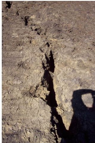
Figure 2: Crack where fill material has fallen into the void
