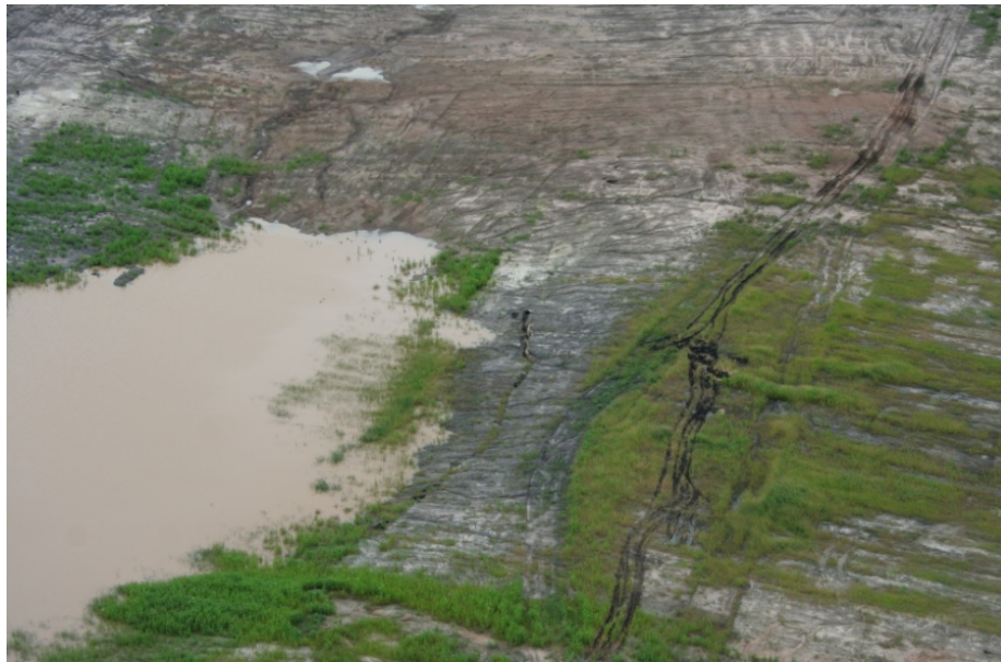
Figure 5: Aerial view of continued crack formation
