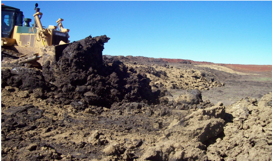
Figure 8: Soil mixing during soil movement
