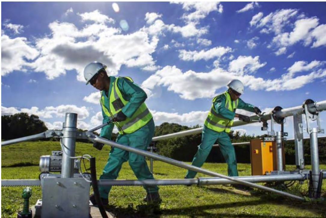
Figure 7: Single Axis Tracking for Panel Mounting
