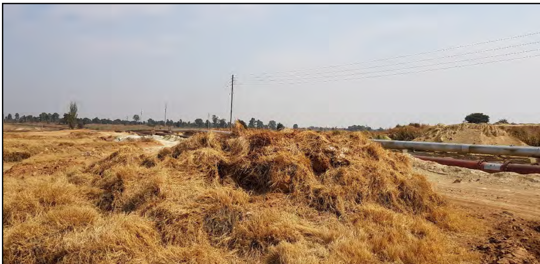
Figure 59: General environment along the slurry pipeline.
