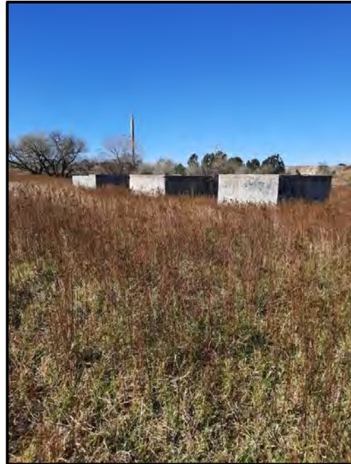
Figure 44: Three small structures at DRD008. The structures are currently occupied by squatters.
