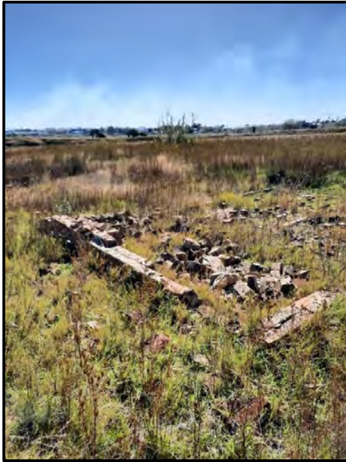
Figure 43: Ruins at DRD007. Only foundations are left in Area B.
