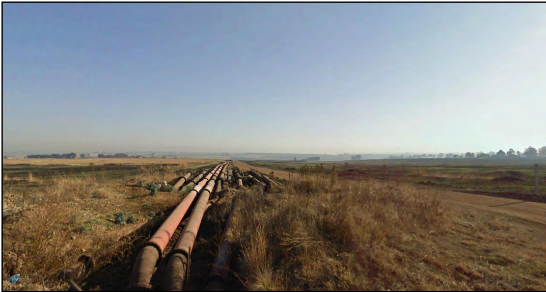
Figure 63: Existing slurry pipeline near the R23 arterial road.
