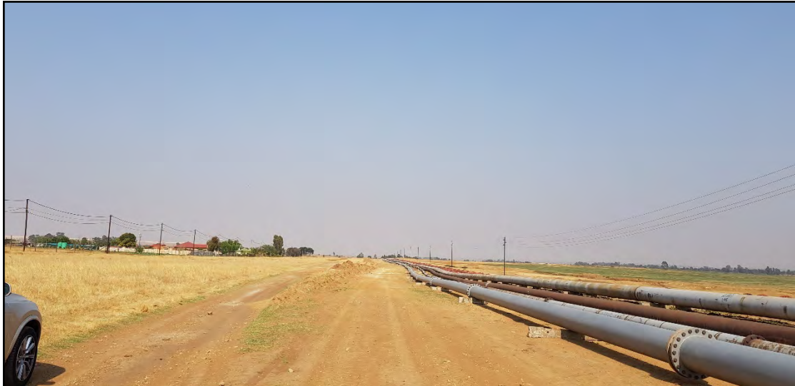
Figure 60: Withok Small Holdings (left) and the proposed Ergo SEF project site (right).
