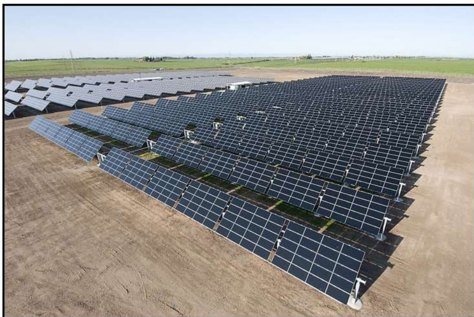
Photographs 5.2.2 and 5.2.3: The photos above and to the right show a typical example of the mounting structure for a tracking PVSEF and an array of photovoltaic panels once mounted
