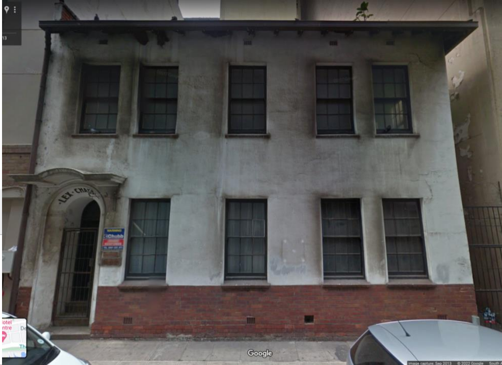
Figure 1: 24 Parry street building
