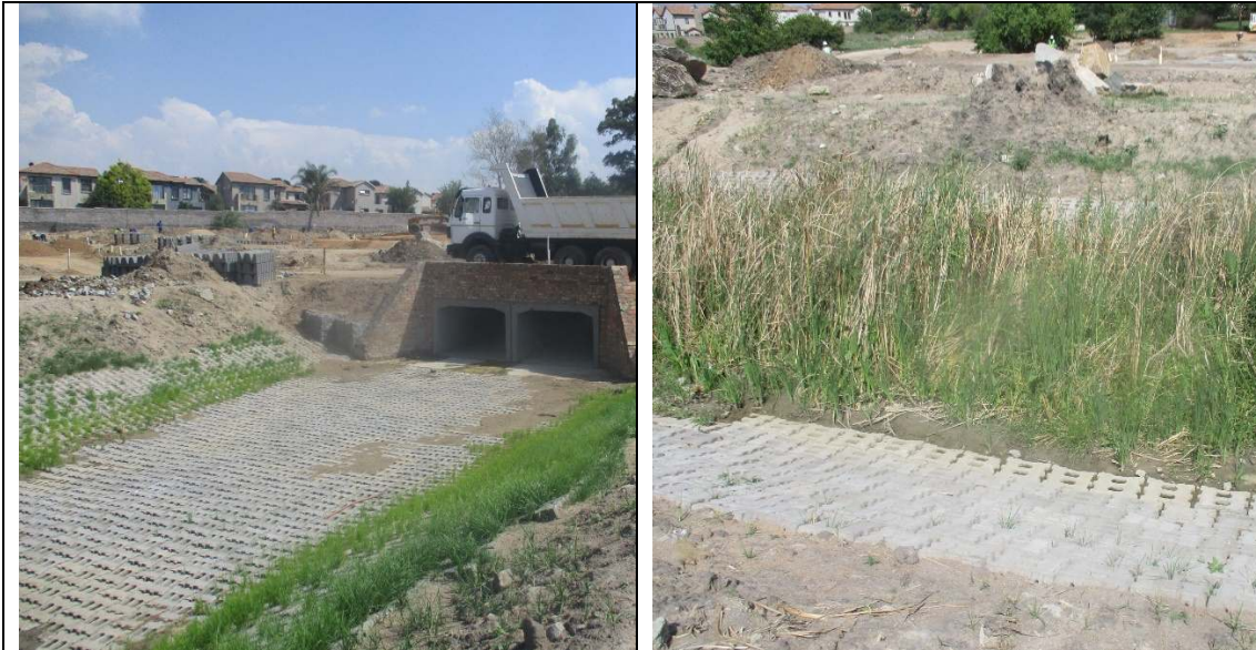
Figure 7: Photograph of armoflex channel on adjacent property
