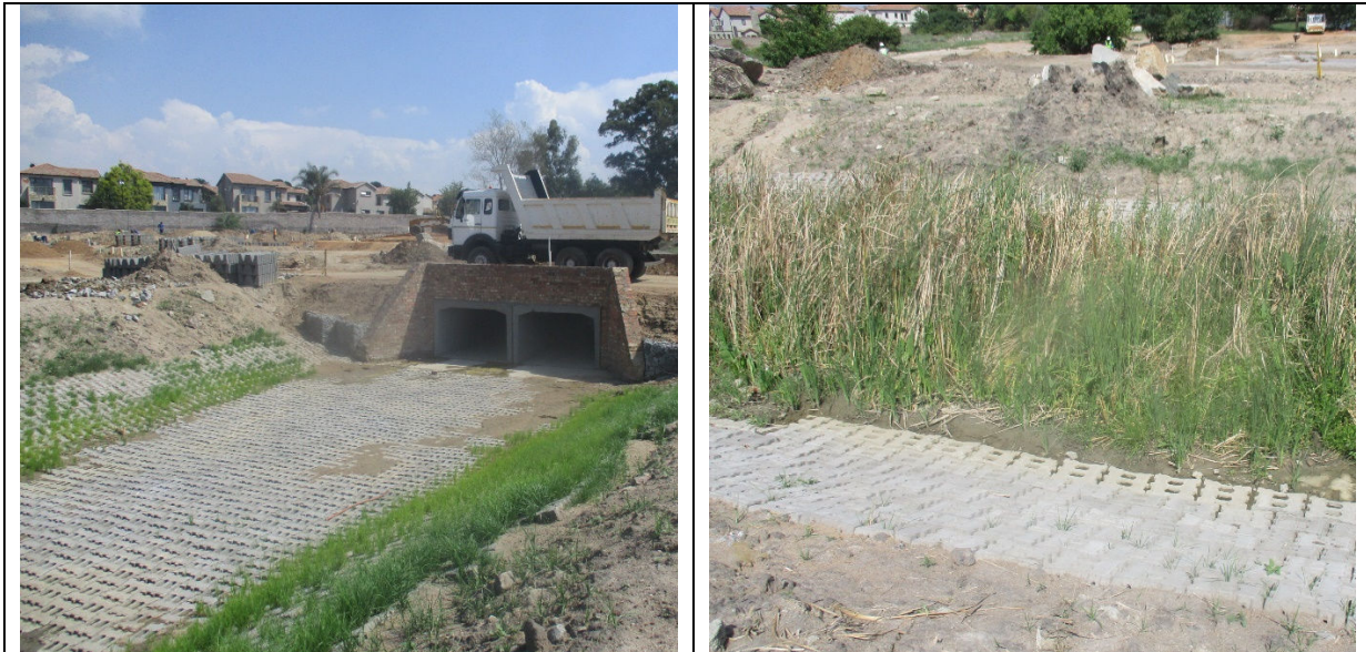
Figure 7: Photograph of armoflex channel on adjacent property
