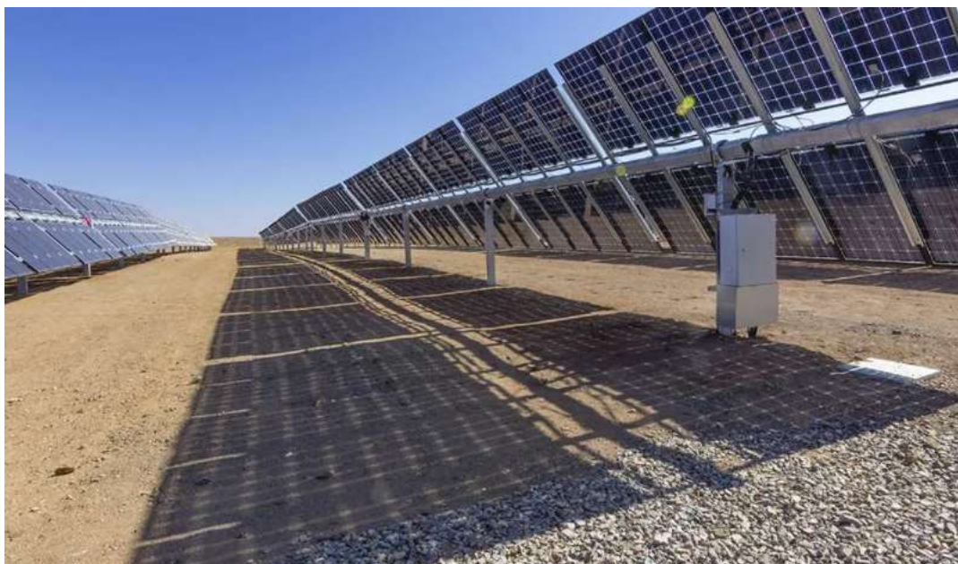
Figure 4: Example of Bi-facial solar panels to be utilised for this project.
