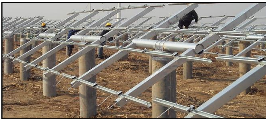
Figure 21: Support structure for Tracking PV Panels
