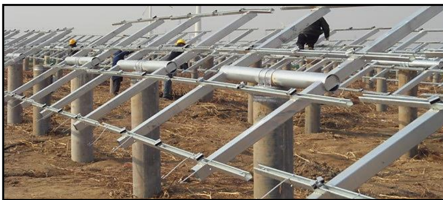
Figure 21: Support structure for Tracking PV Panels
