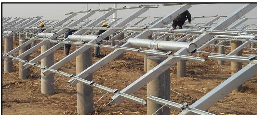
Figure 21: Support structure for Tracking PV Panels
