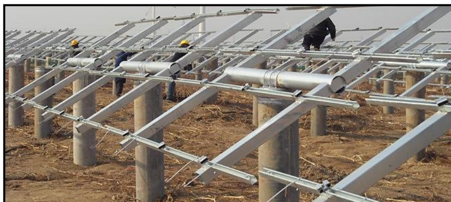
Figure 21: Support structure for Tracking PV Panels
