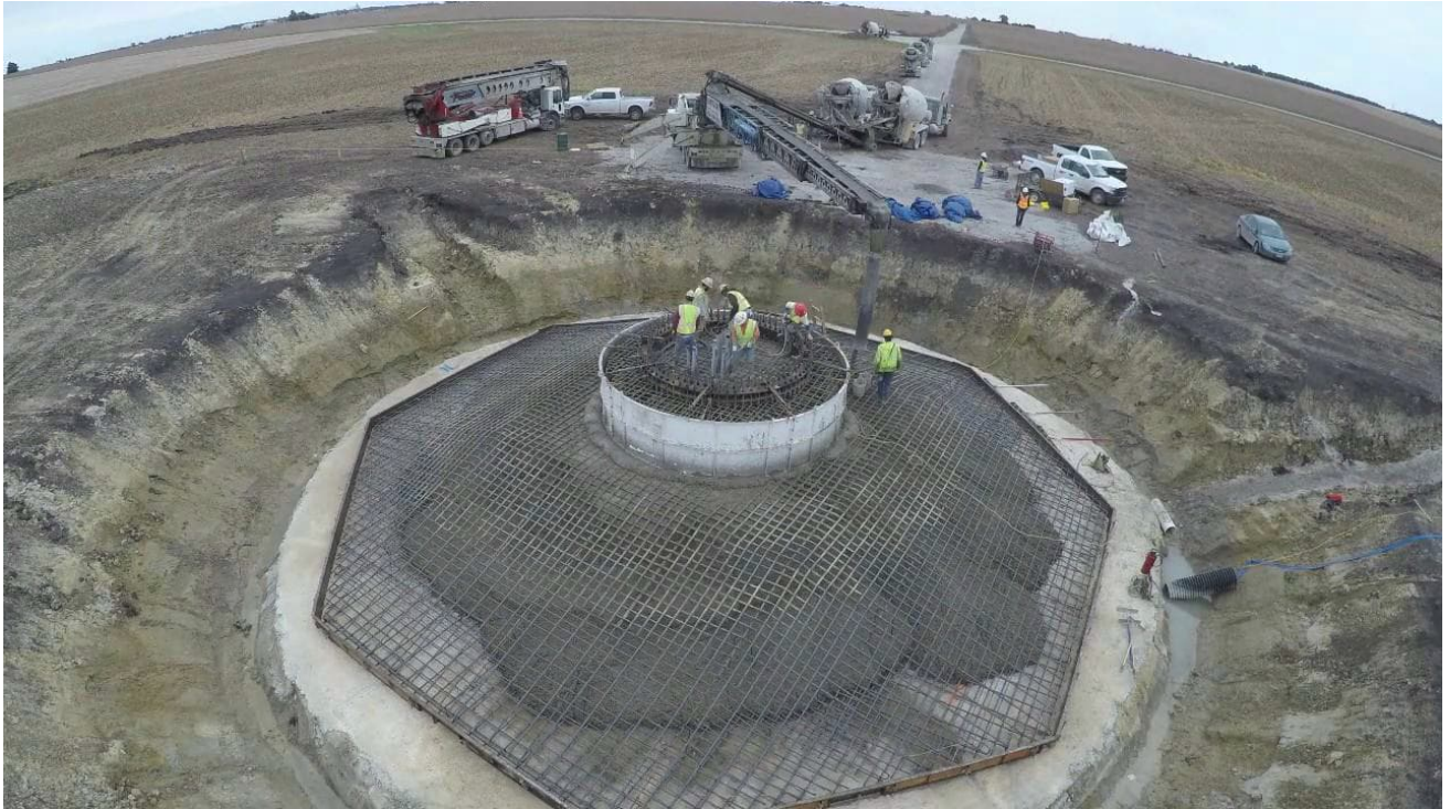
Figure 6-1 - Typical Wind Turbine Foundation Construction. Image source: Kevin, 0:23
