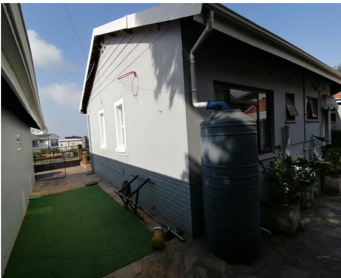
REAR OF HOUSE AND RIGHT SIDE
