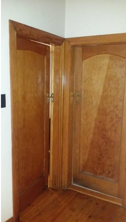
Previous Toilet and bath converted to guest Toilet and Shower (Frames and doors stripped and restored)
