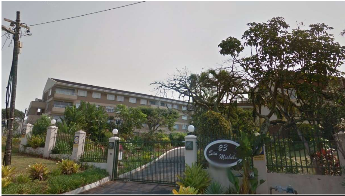
PHOTO 10 – CONTEXUAL PHOTO OF THE ENTRANCE AND AJACENT BUILDING
