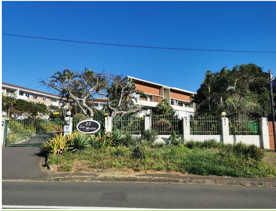
PHOTO 01 – VIEW OF THE ENTRANCE FROM NORTH EAST (PARK DRIVE SIDE)
