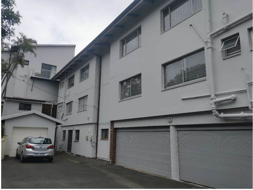
PHOTO 05 – VIEW FROM THE SOUTH EAST - ADJACENT UNIT 02 AND APARTMENTS
