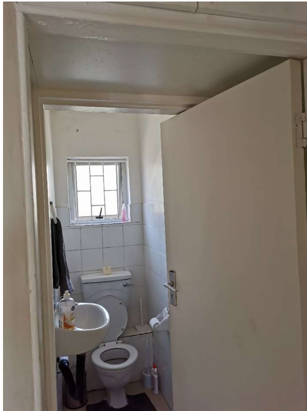
PHOTO 09 – VIEW OF THE EXISTING TOILET TO BE REFURBISHED
