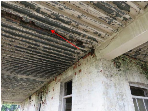
Photo 27: Collapsing Roof and Ceiling Structure
