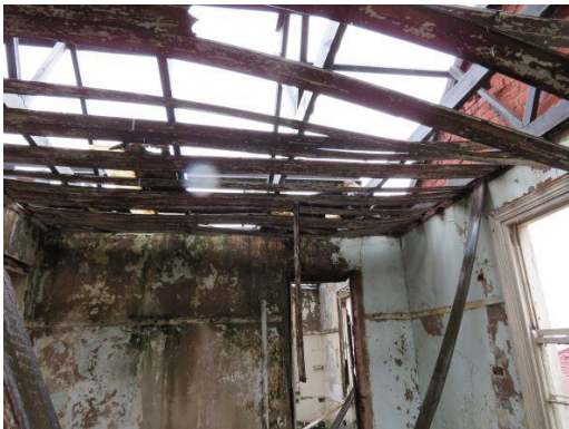
Photo 27: Collapsing Roof and Ceiling Structure
