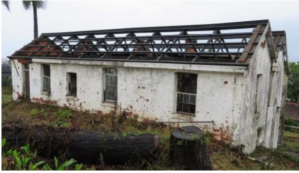
Photo 25: Bare roof structure without roof sheeting
