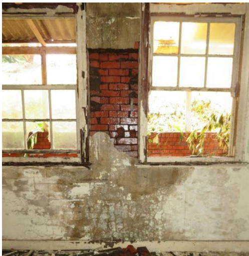
Photo 13: Water damage to basement walls
