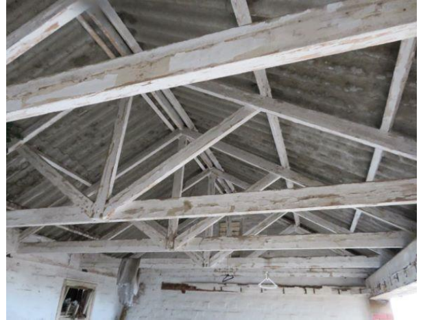
Fig 8: Internal View of Block C
