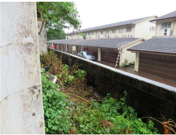
Photo 69: Retaining wall at the lower boundary of the site
