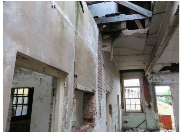
Fig 4: Typical Interior View Block A
