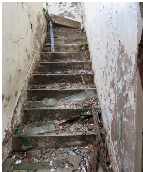
Photo 41: Stairs to 1 st Floor Level
