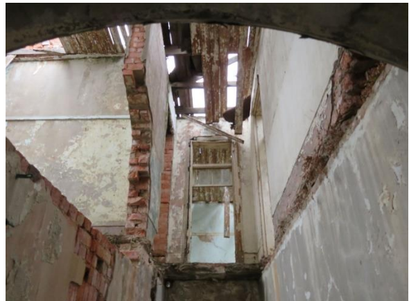
Fig 6: Internal View of Block B
