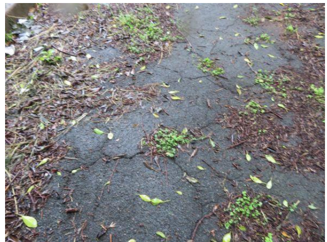
Photo 64: Typical Driveway Surfacing Condition
