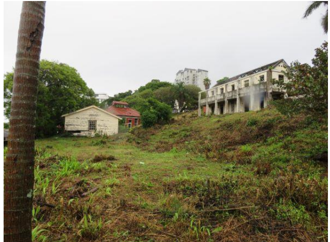
Photo 70: Typical View of site from the North Eastern Side
