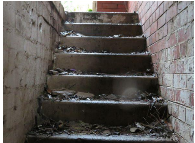
Photo 22: Stairs to Basement
