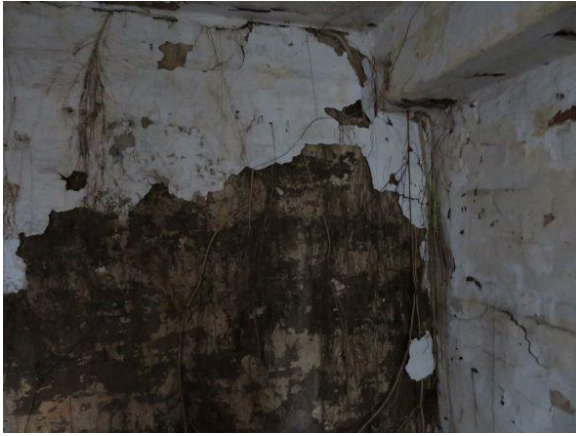
Photo 13: Water damage to basement walls
