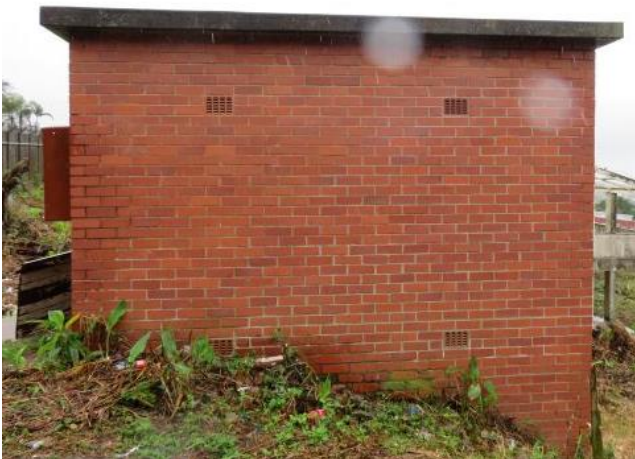
Photo 51: Typical Brick Wall Condition (fairly good)
