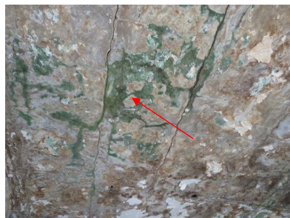
Photo 34: Very Poor Condition of RC Slab Soffit Signs of Cracks and Water Ingress through Slab
