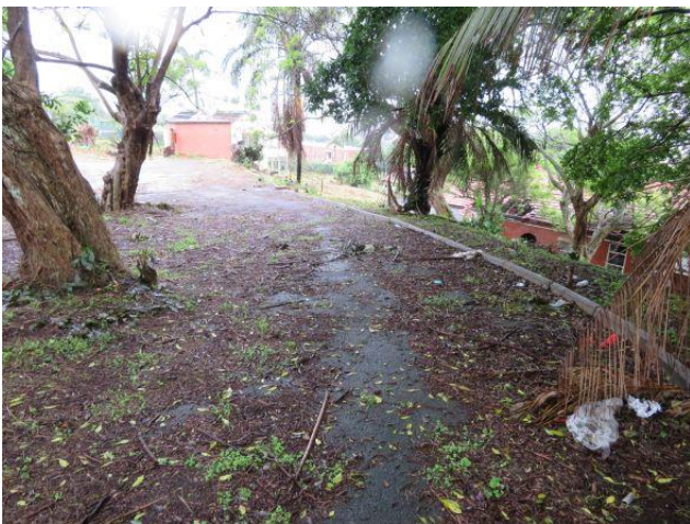
Photo 63: Typical Driveway Condition
