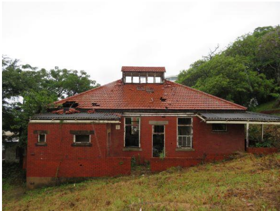
Fig 3: External View of Main Block A
