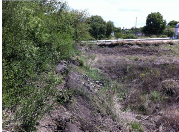
Looking South of Tar Dam D
