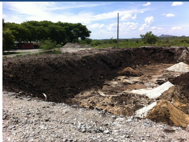
Looking North West of Tar Dam A
