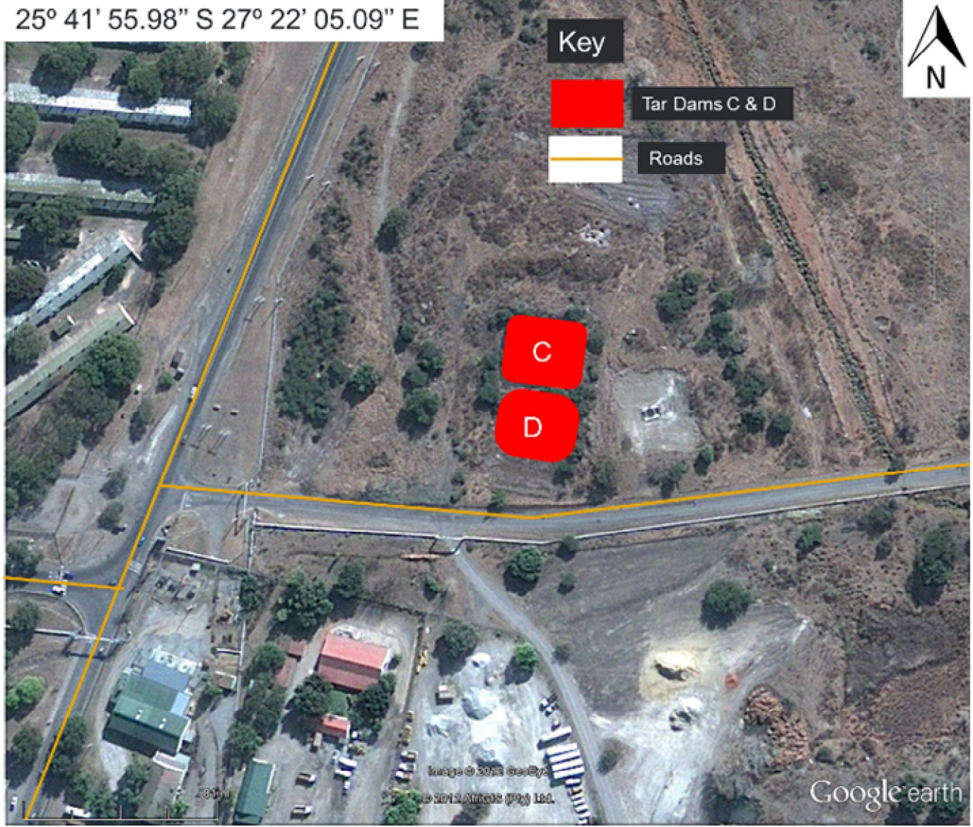
FIGURE 2: Tar Dams C and D (Source: Google Earth 2012)
