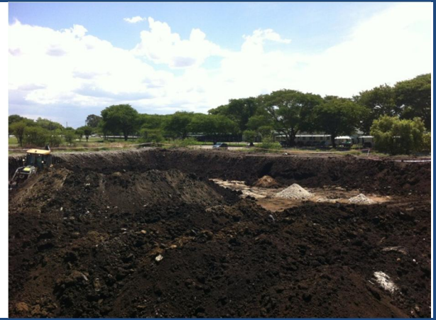
South West of Tar Dam A
