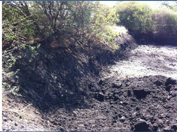
Looking South West of Tar Dam C
