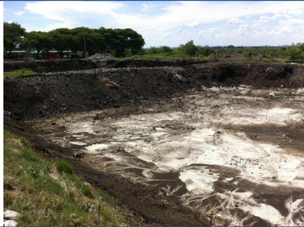
Looking North West of Tar Dam B
