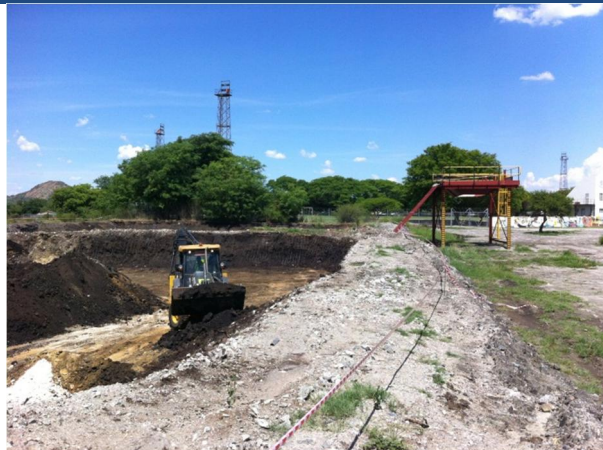
Looking East of Tar Dams A and B
