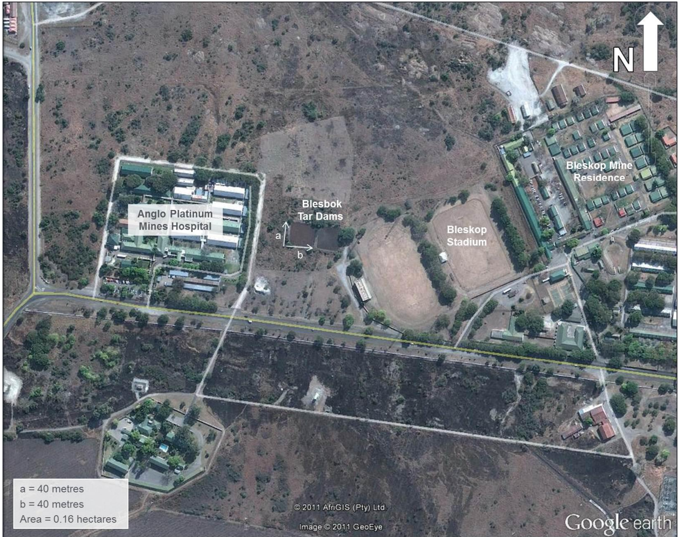
Figure 2: Aerial Image illustrating Tar Dams A and B (Source: Google Earth, 2012)
