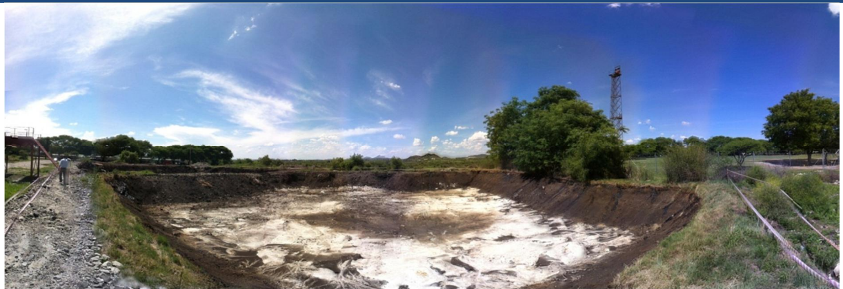
Looking from the West to the North East of Tar Dams A and B (Tar Dam B in foreground)
