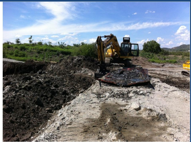
Looking North of Tar Dam C
