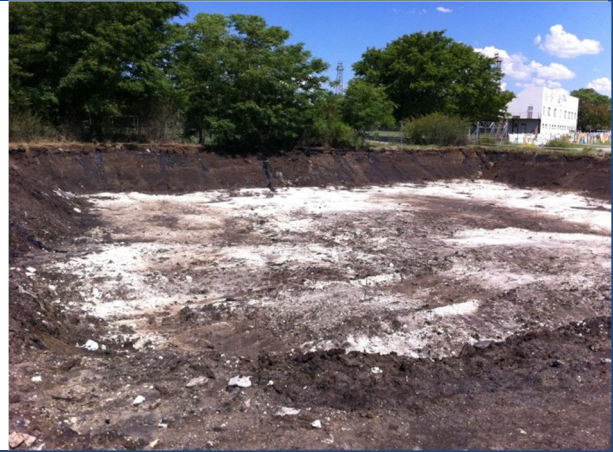
Looking South East of Tar Dam B
