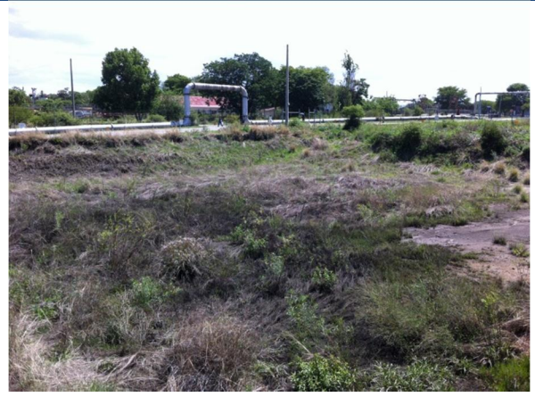
Looking South West of Tar Dam D
