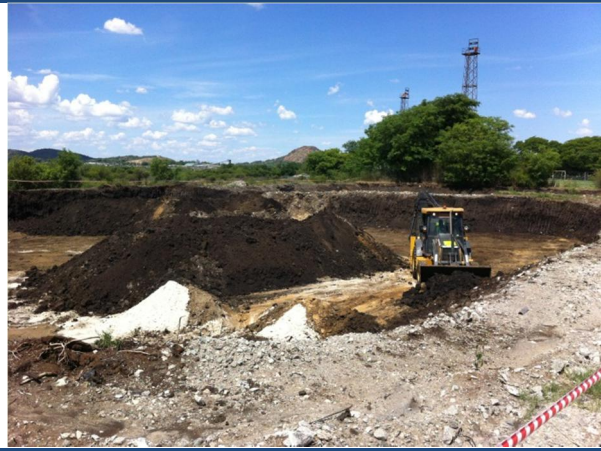
North East of Tar Dam A
