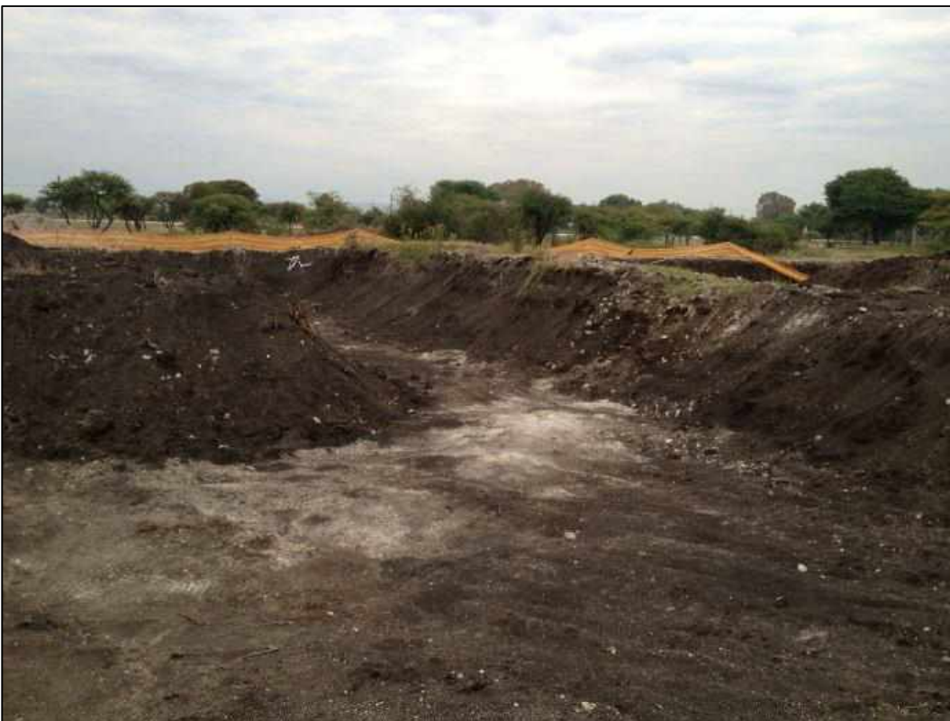
Plate 3. View of decommissioning works (South West)
