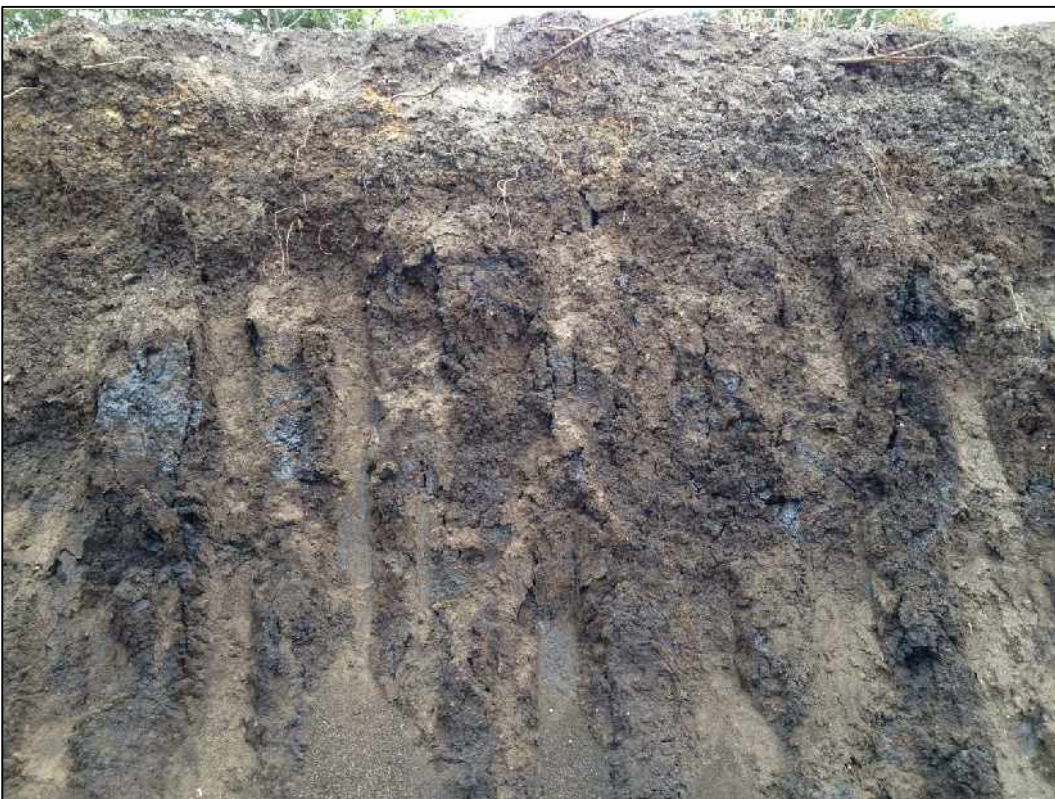
Plate 11. View of tar residue seeping out of pit wall on Tar Dam A (West)
