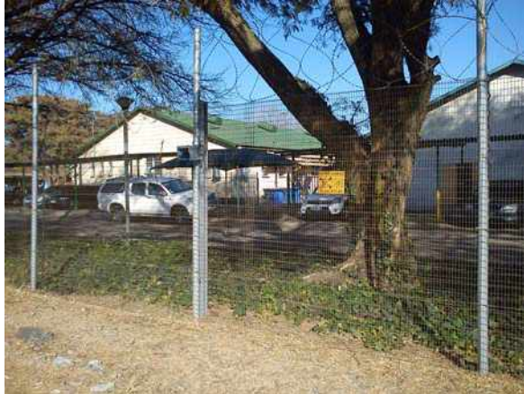
Photo No 1: Location 1 (Anglo Plat Medical Centre Eastern fenceline)
