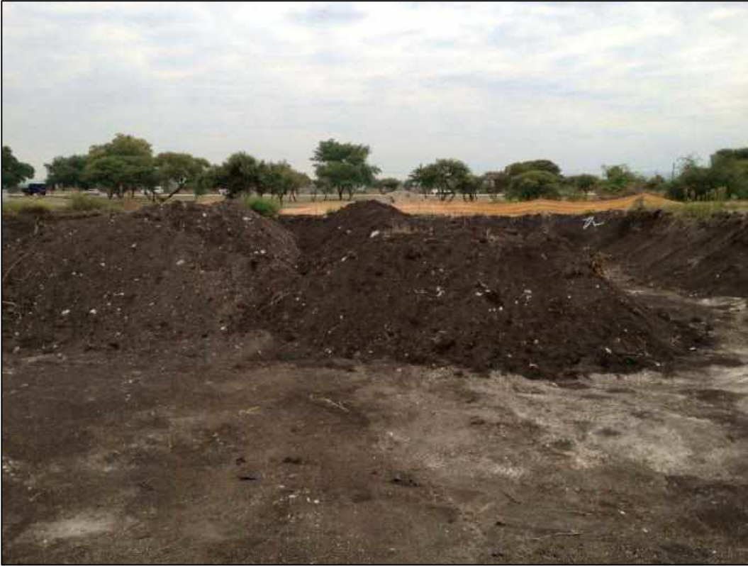
Plate 2. View of decommissioning works and excavated material (South)
