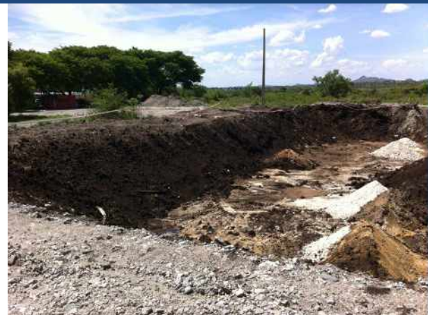
Looking North of Tar Dam A
