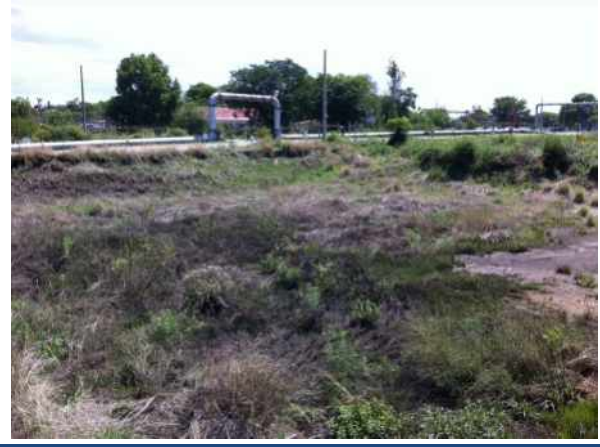
Looking South West of Tar Dam D
