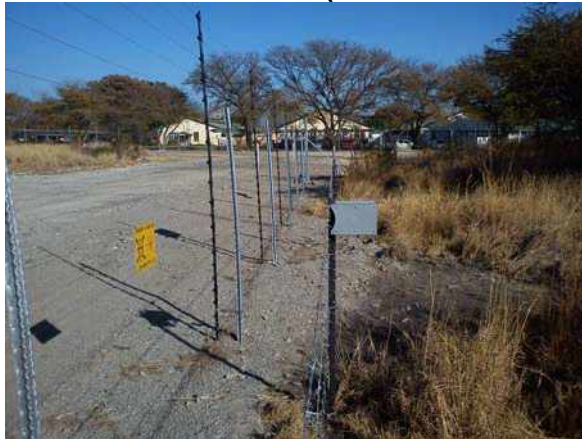
Photo No 2: Location 2 (Southern dam wall)
