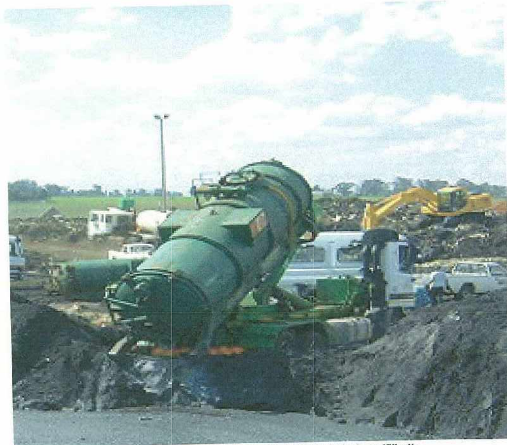
Photograph 10: Disposal at Holfontein Landfill site
