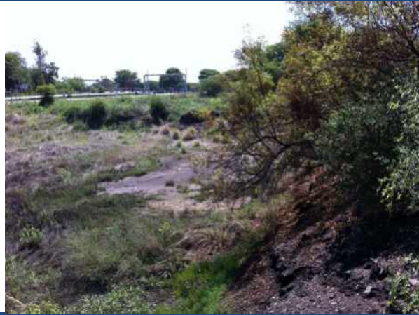
Looking West of Tar Dam D
