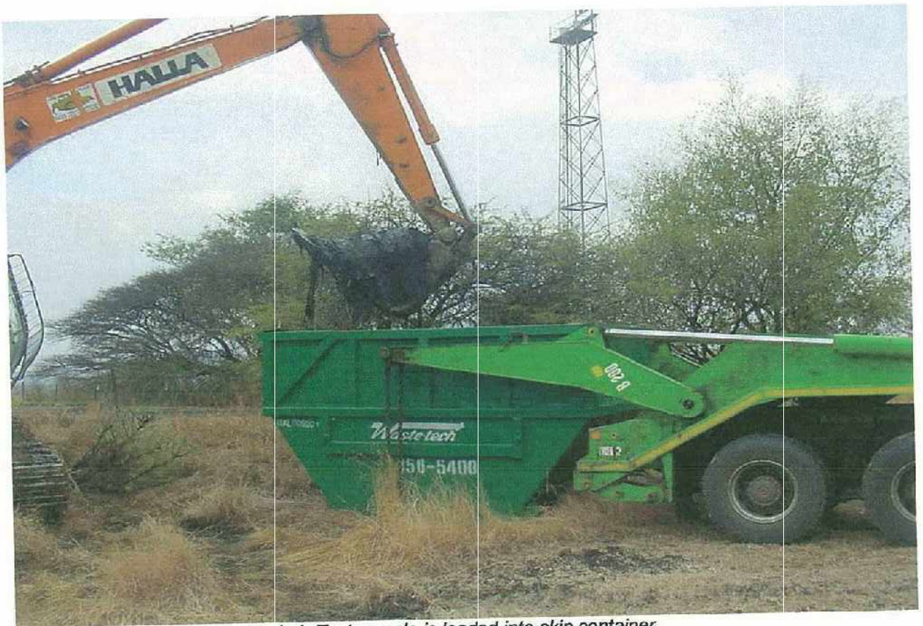
Photograph 4: Test sample is loaded into skip container
