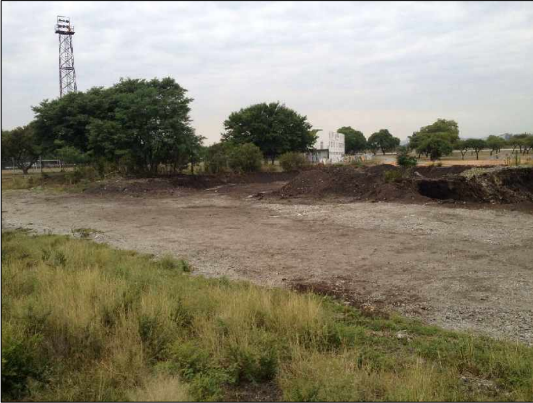
Plate 6. View of decommissioning works on Tar Dam B (south East)
