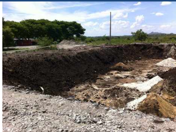
Looking North West of Tar Dam A
