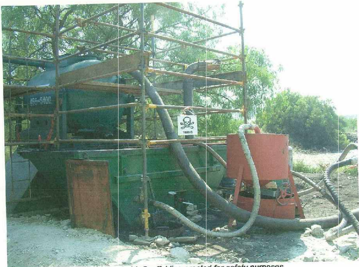
Photograph 14: Scaffolding erected for safety purposes
