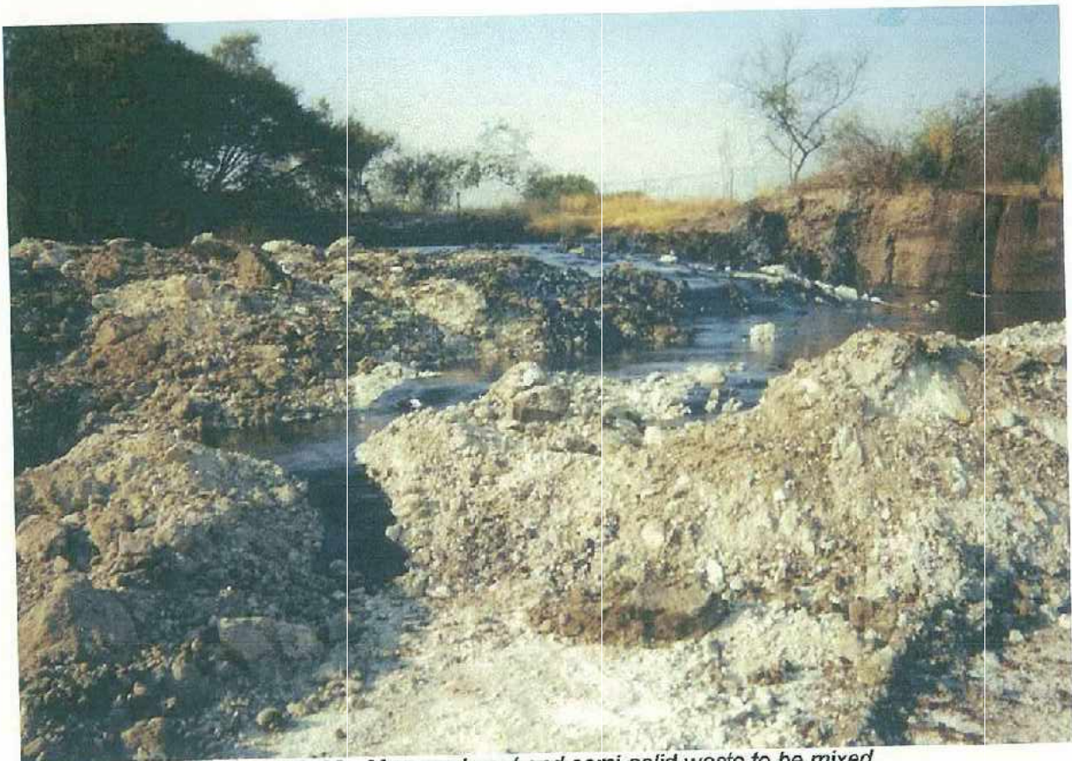
Photograph 23: More undercut and semi-solid waste to be mixed
