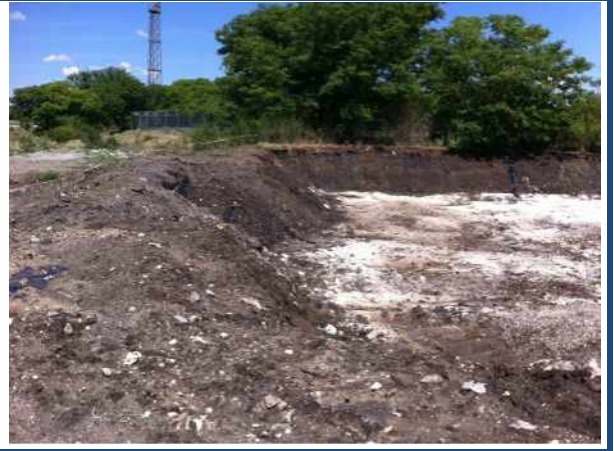
Looking East of Tar Dam B
