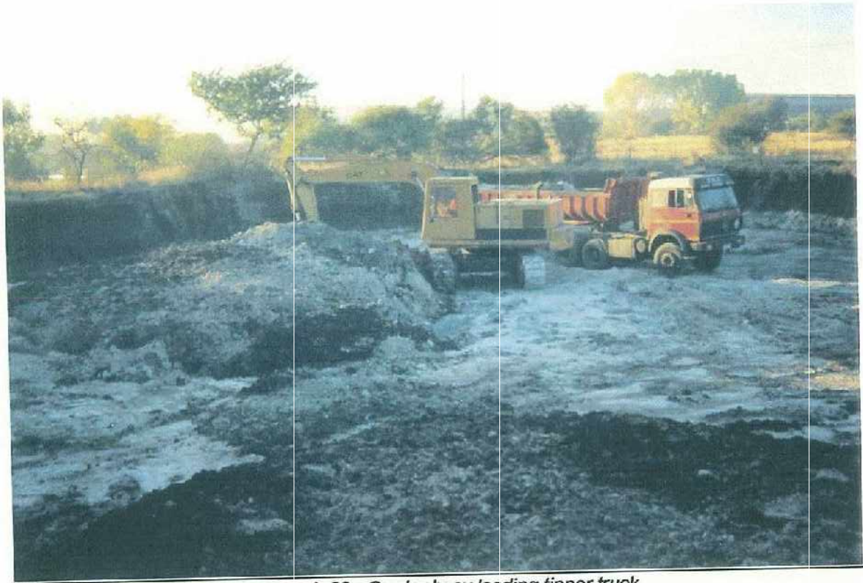
Photograph 22: Grader busy loading tipper truck
