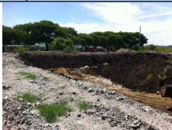
Looking West of Tar Dam A
