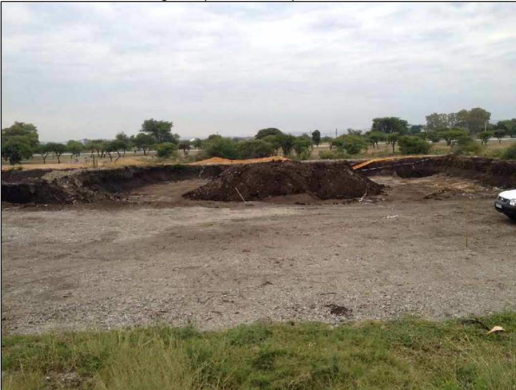
Plate 5. View of decommissioning works on Tar Dam A (South)
