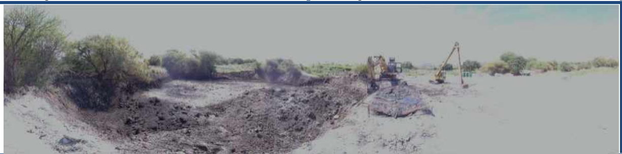
Looking from the North East to the West of Tar Dam C
