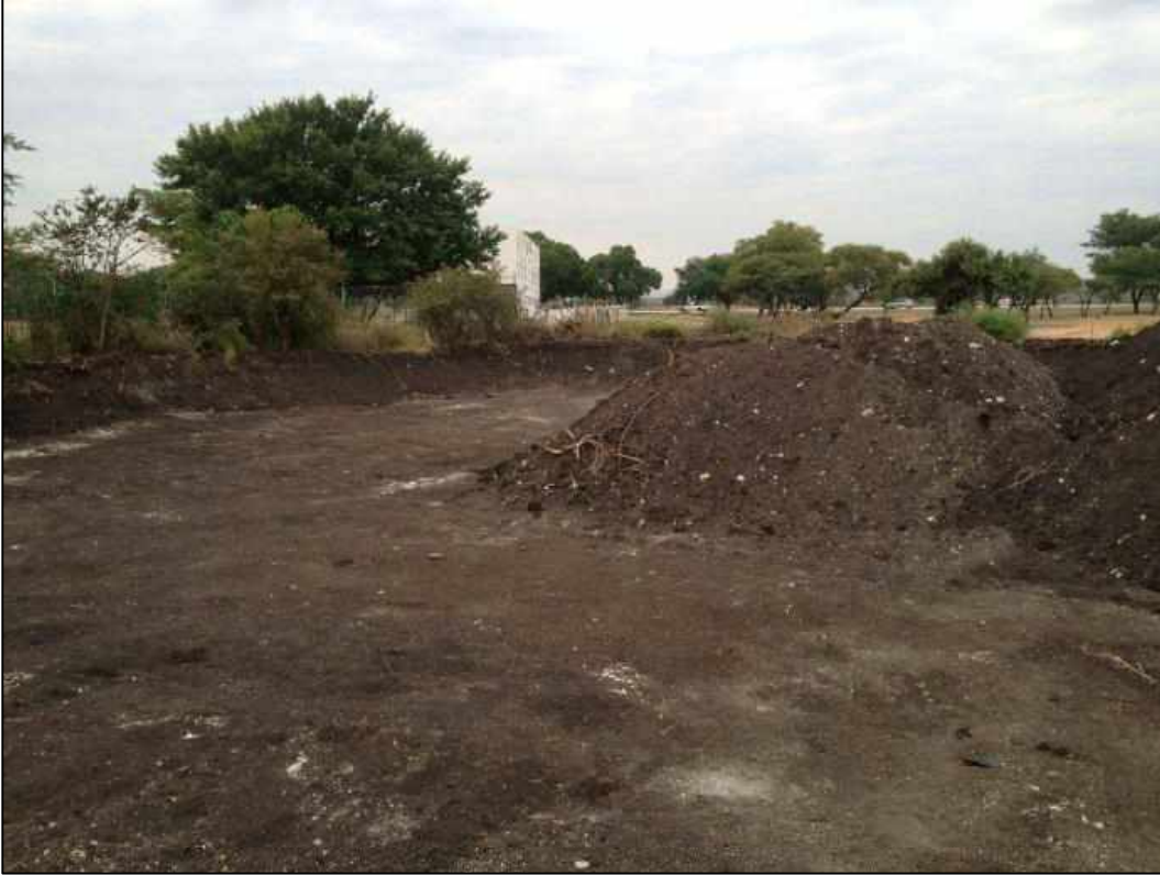
Plate 1. View of decommissioning works (South East)
