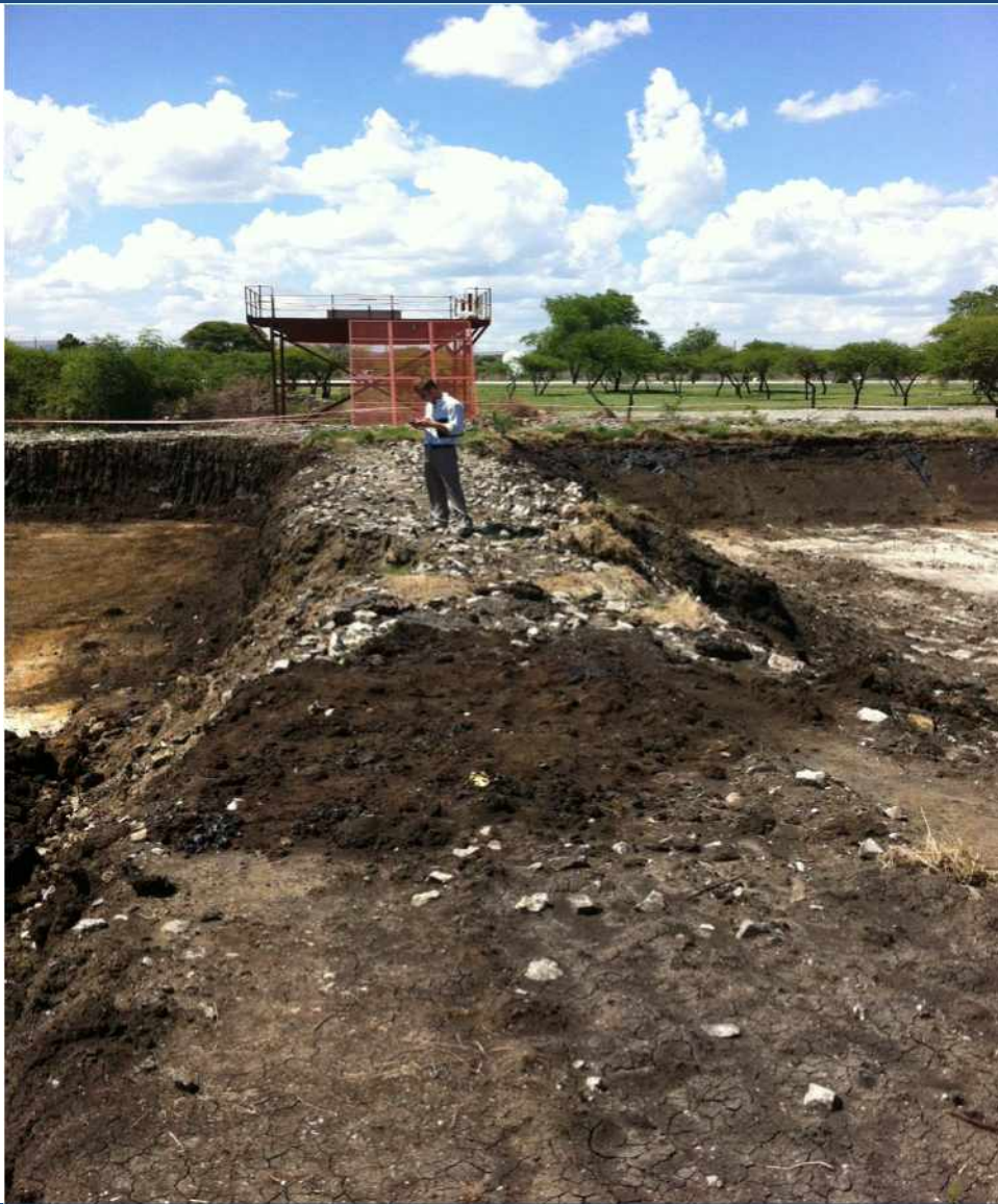
Looking South of Tar Dams A and B
