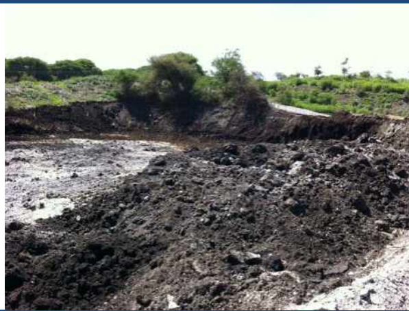
Looking North West of Tar Dam C
