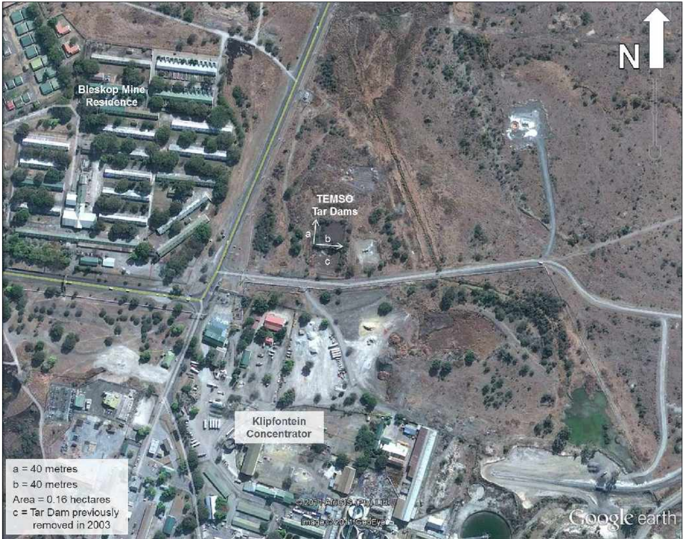
Figure 3: Aerial Image illustrating Tar Dams C and C (Source: Google Earth, 2012)
