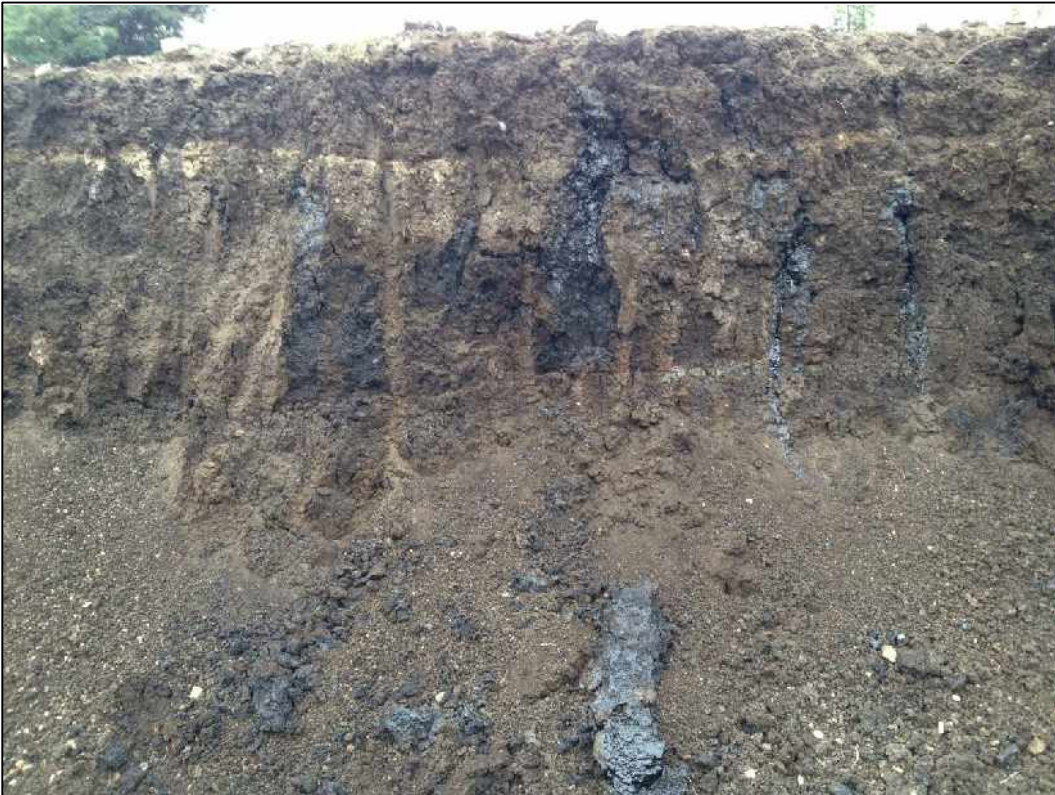
Plate 7. View of tar residue seeping out of pit wall on Tar Dam B (East)
