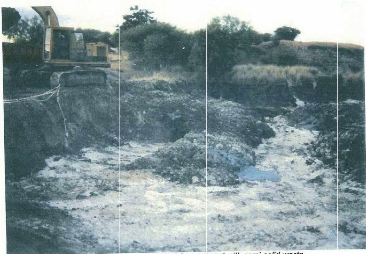
Photograph 21: Grader busy mixing undercut with semi-solid waste
