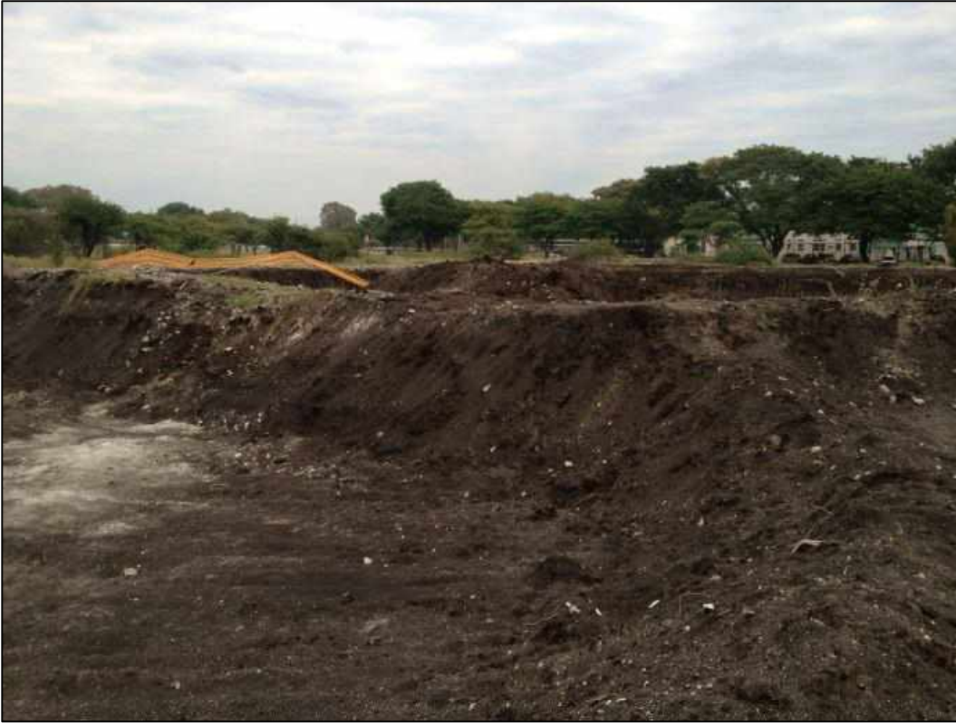
Plate 4. View of decommissioning works (West South West)
