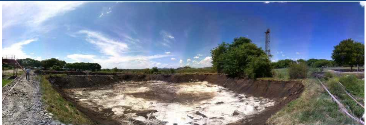
Looking from the West to the North East of Tar Dams A and B (Tar Dam B in foreground)
