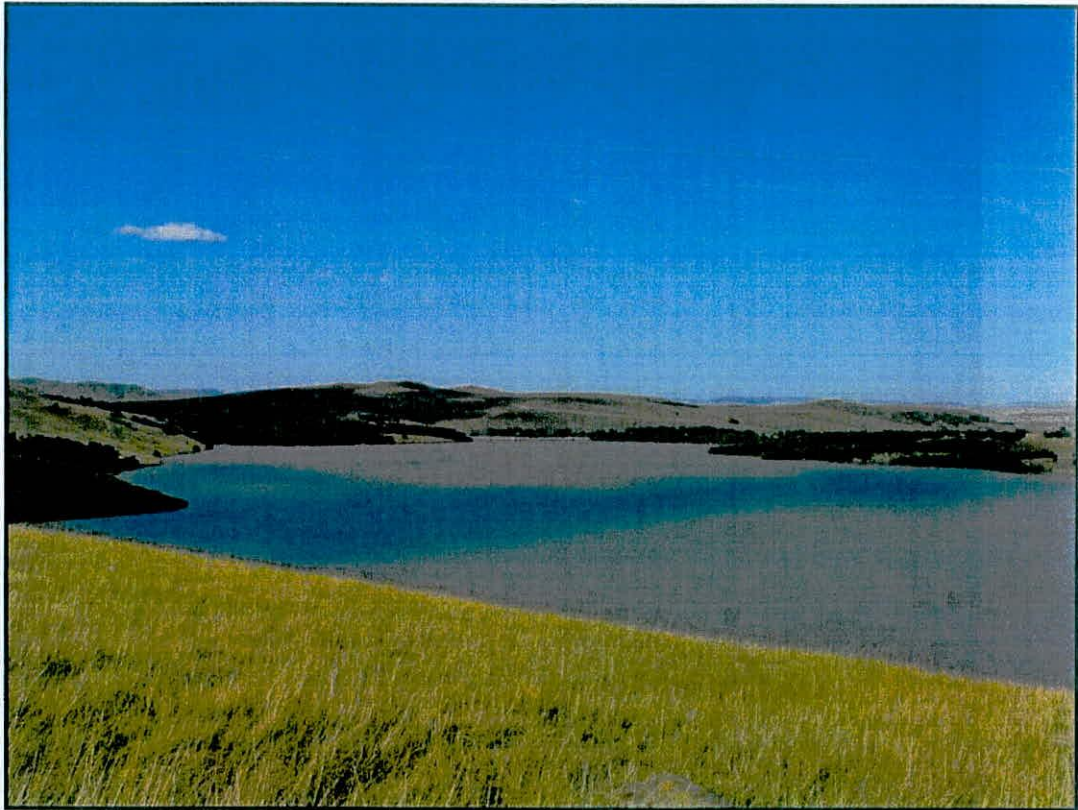
Fig. 7. Looking east towards the dam wall.
