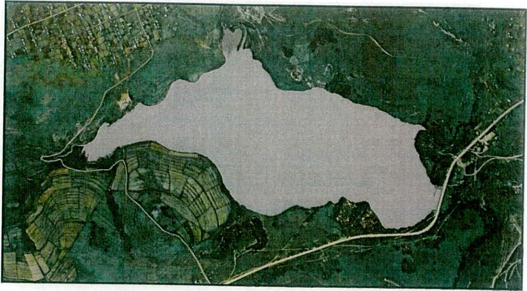
Fig. 4. Aerial photograph of the dam. (Photo: Google Earth)
