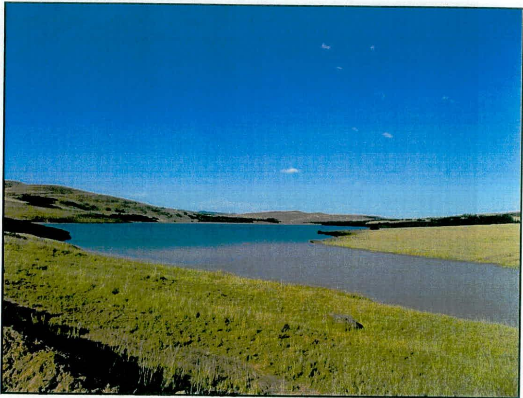
Fig. 6. Looking west, upstream of the dam wall.
