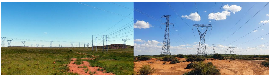
Figure 2: Several existing power lines traverse the area (with associated disturbed areas such as access track and cleared servitudes already existing below the lines). The proposed power line route considered in this proposal follows existing power lines for the majority of its route.
