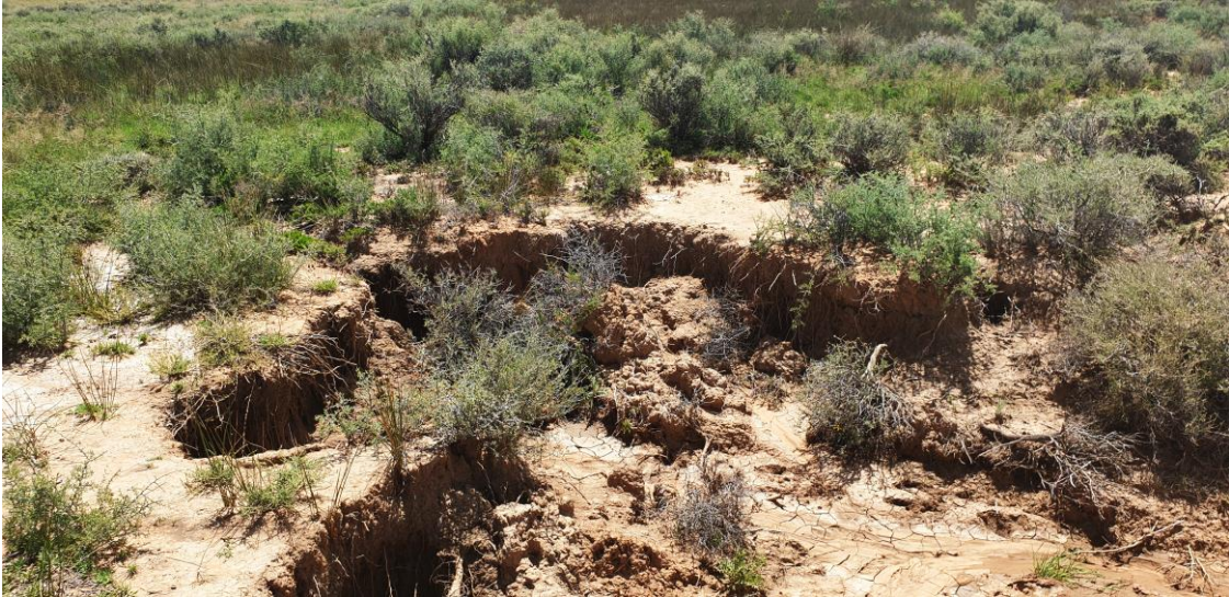
Figure 13: Erosion is occurring in multiple areas along the existing power line servitude, the existing servitudes that are to be utilised must be upgraded with effective erosion control measures to prevent further degradation of habitat.
