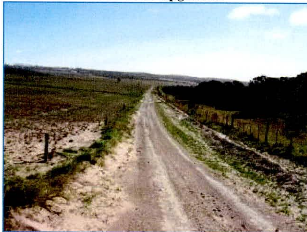
Access road to be upgraded
