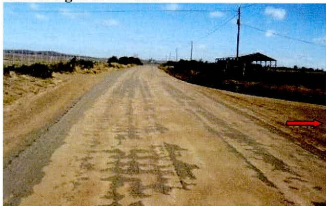
Line of sight to the east
