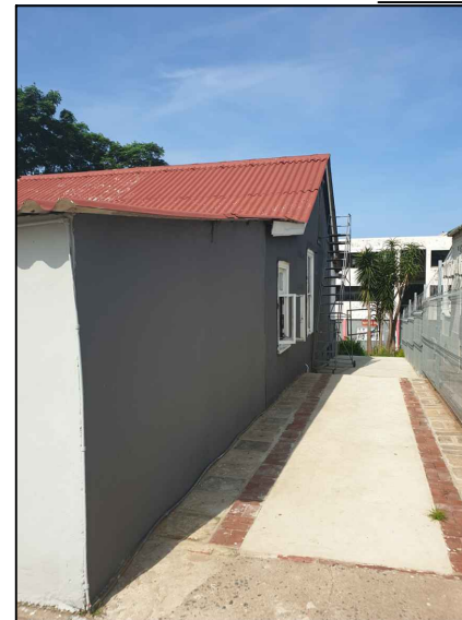
South Facing Side of House
