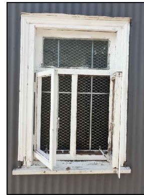
Window on South side
