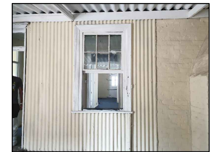
West Facing inside back of enclosed area (Rear)
