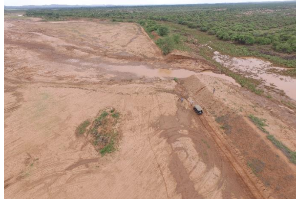
View of bund-wall and path of destruction
