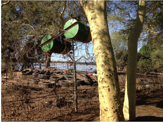
Extraction point damaged by flood waters
