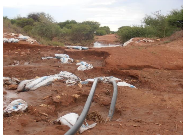
Damage on Weipe road and irrigation pipes
