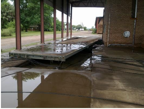
Weighbridge lifted out of housing
