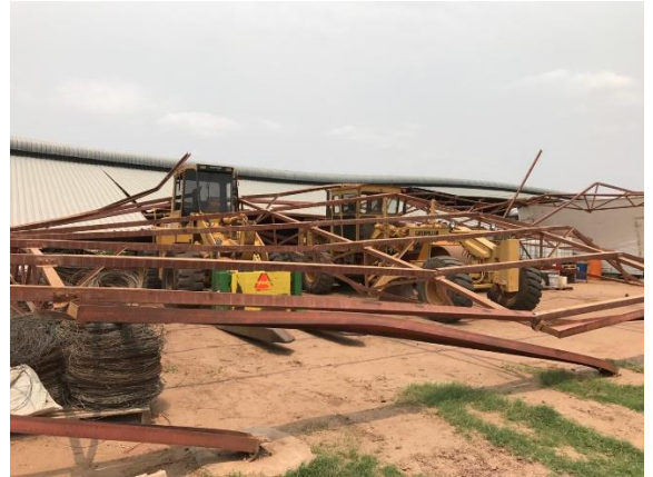
Equipment under collapsed shed (roofing ripped of)
